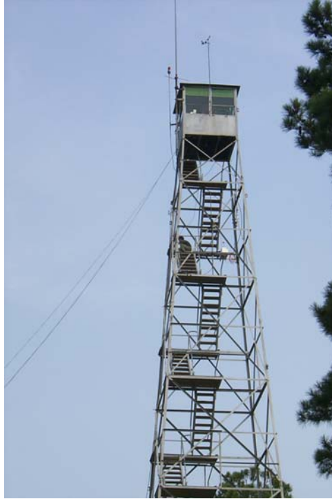
Figure 3.1. Typical Fire Tower with Staff Working at Upper Sampler Height
