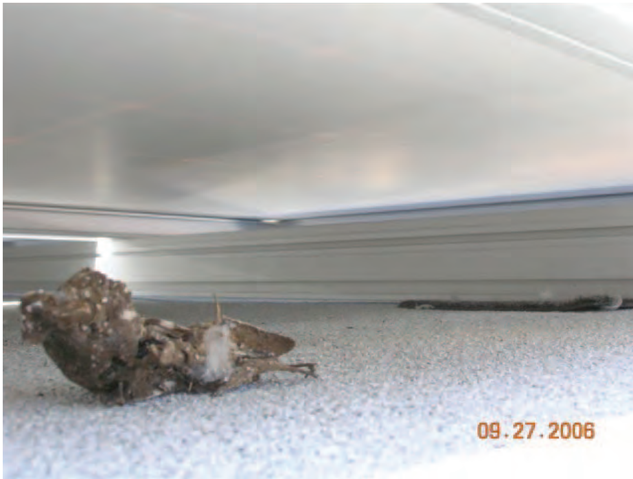
Photo #2 Rat thought to have been electrocuted while chewing on PV module wiring (J. Wiles)
