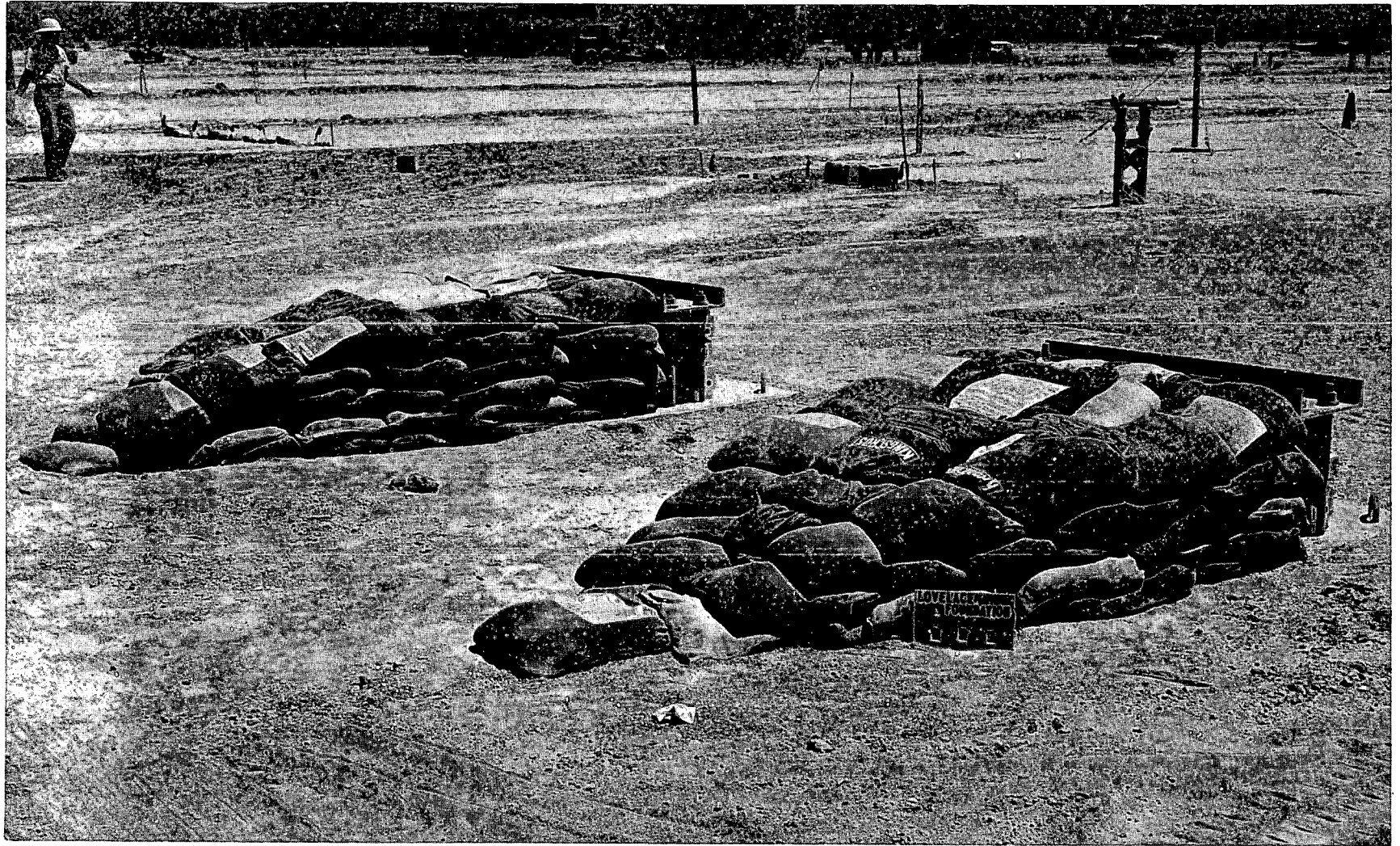
Fig. 4.134—Installations 15P3 and 15P4, preshot.
