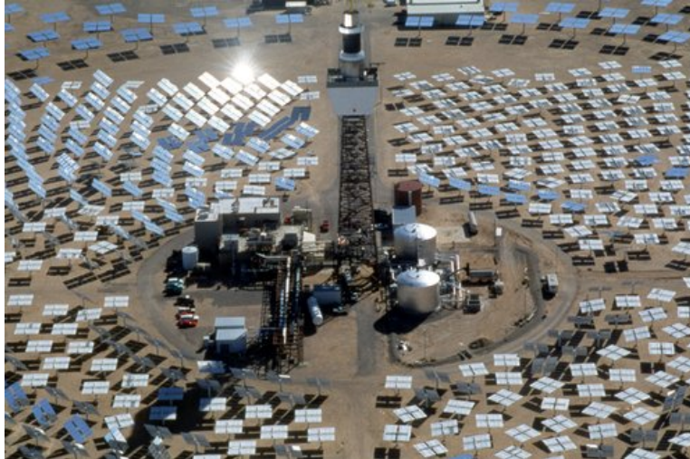
Figure 3-32 Solar Power Tower Collector, Solar Two at Daguerre, California (Source: NREL 2012d)
