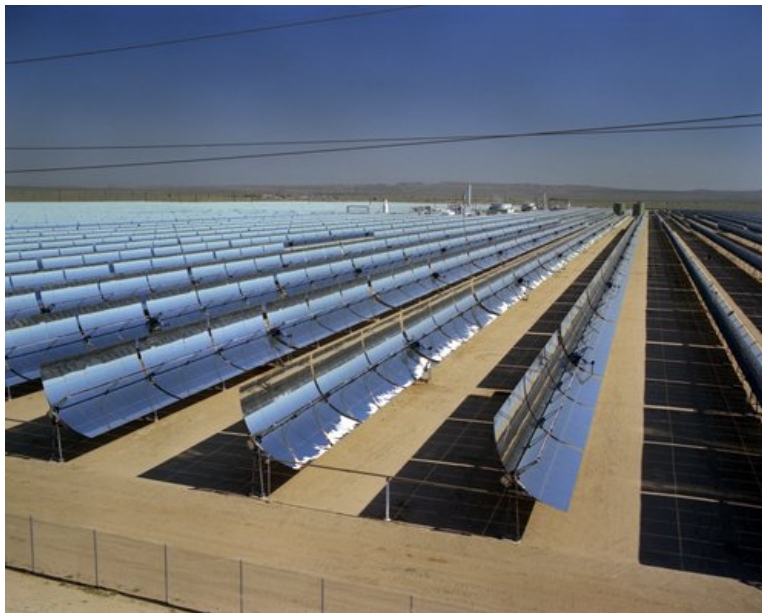
Figure 3-31 Parabolic Trough Concentrating Solar Collector at Kramer Junction, California (Source: NREL 2012c)
