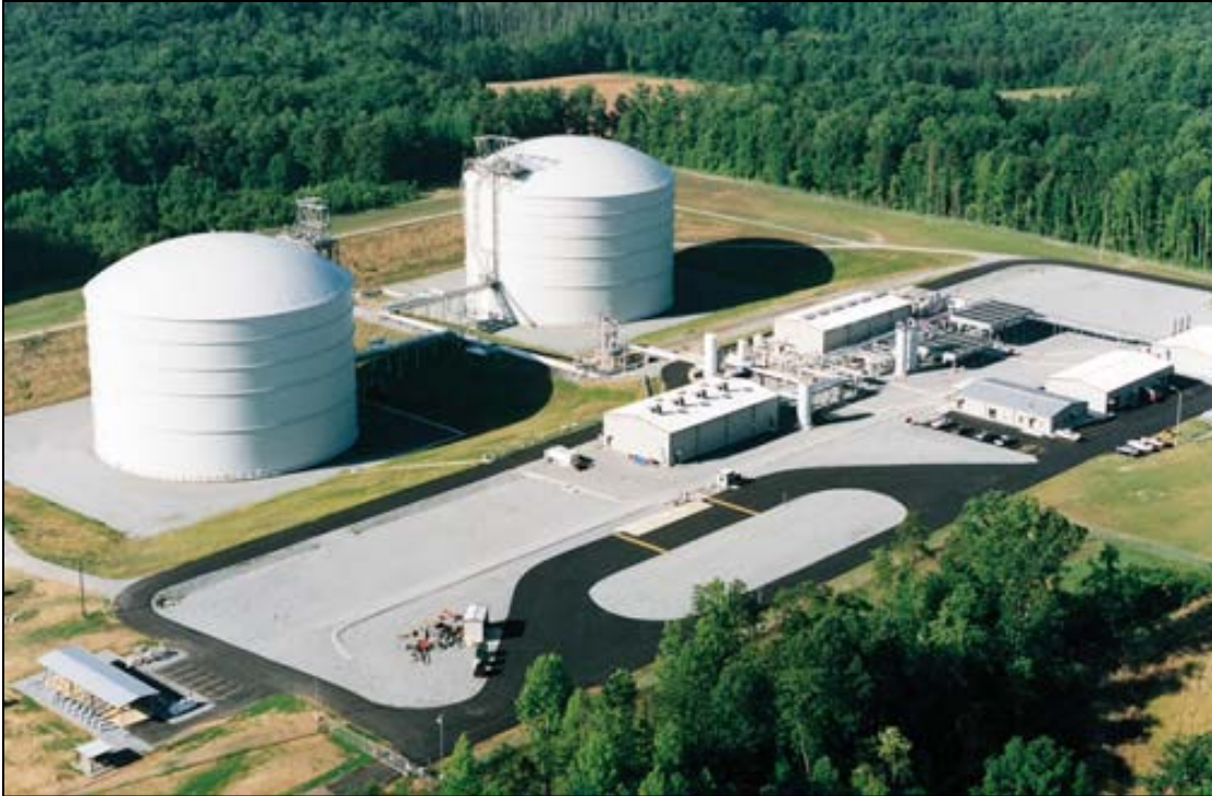
Figure 3-20 LNG Storage and Peak Shaving Facility (Source: DOE 2005)
