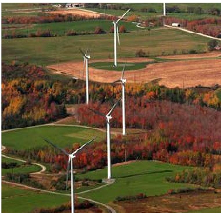
Figure 3-42 Maple Ridge Wind Farm in Lewis County, New York (Note: The wind farm contains a total of 195 1.65-MW wind turbines.) (Source: NREL 2013)
