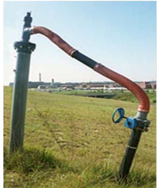
Figure 41. Landfill gas collection well head. The wells have perforated pipes at the bottom and can be 100 feet deep or more.
