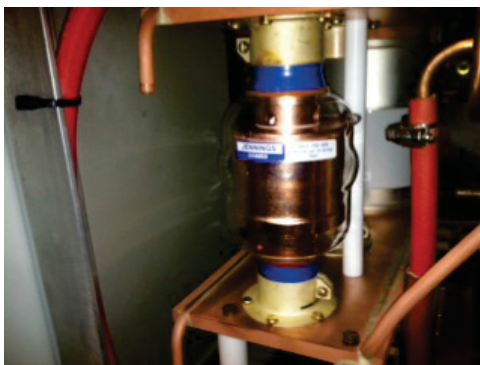
Figure 149. New variable capacitor to replace one of two fixed capacitors.
