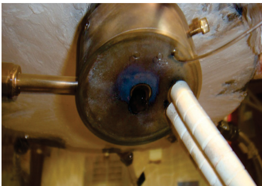
Figure 141. CCIM Drain Assembly as viewed from below the melter.
