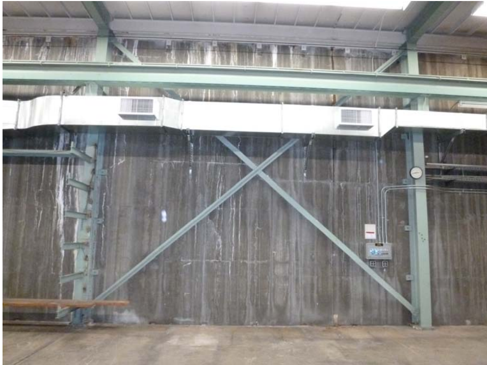
Figure 10 – Increment 2 Tension Only Bracing
