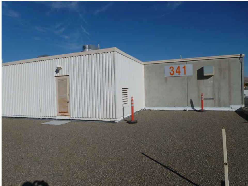
Figure 7 – Southwest Corner of Mechanical Room
