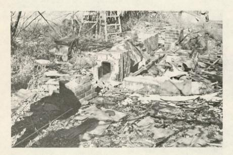
Photo #21: Station #5, collapsed chimney after several pull tests.
