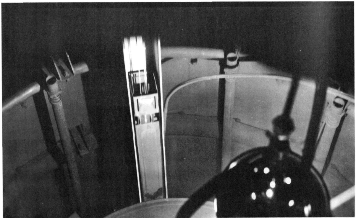
Figure 6. EBWR Core-I Fuel Element Mounted in Submerged Rack Inside Reactor Vessel. (Probe can be seen entering channel.)
