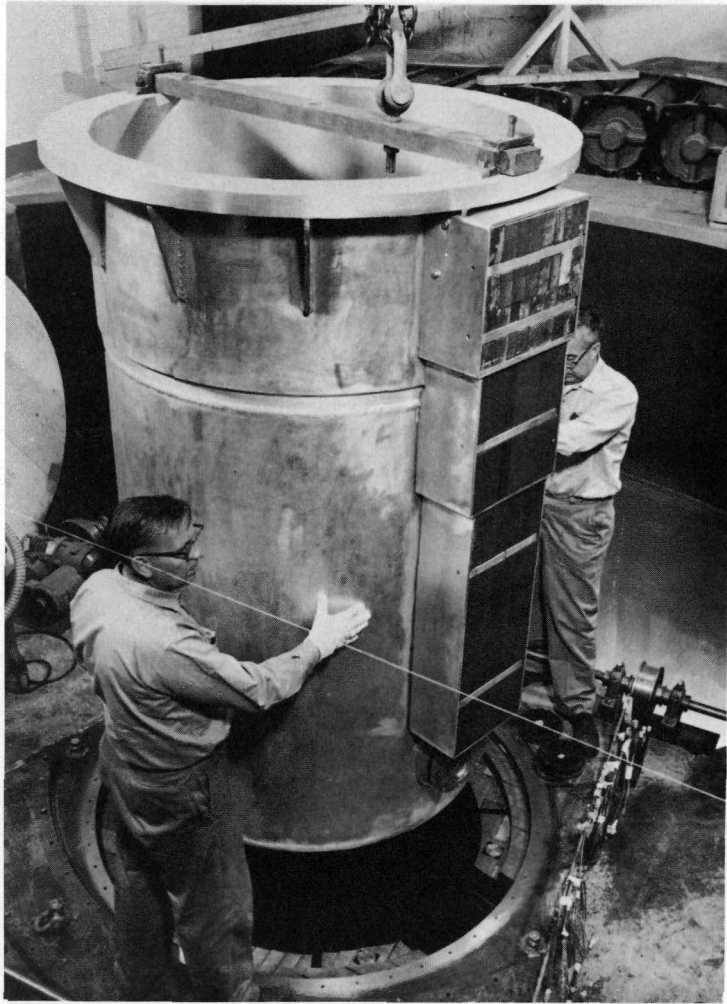
Fig. 20. Reactor Tank and Attached Stepped Section of Graphite System Poised for Insertion
