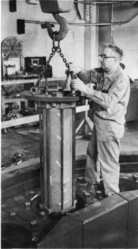
Fig. 51. Pneumatic Cylinder and Shielding Support for "Janus" Shutter
