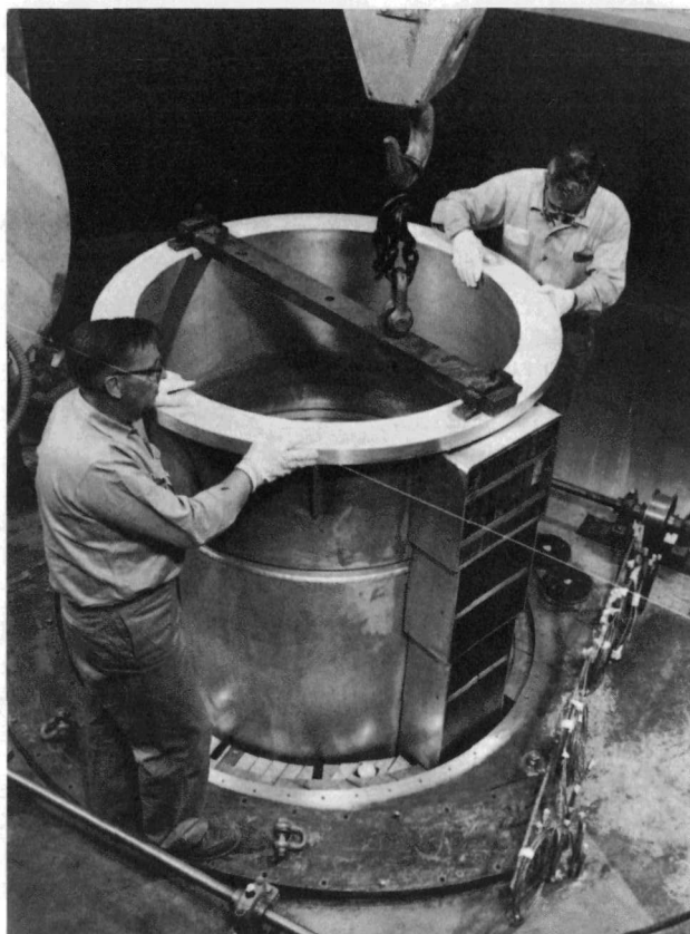
Fig. 36. Reactor Tank Partly Inserted in Principal Graphite System
