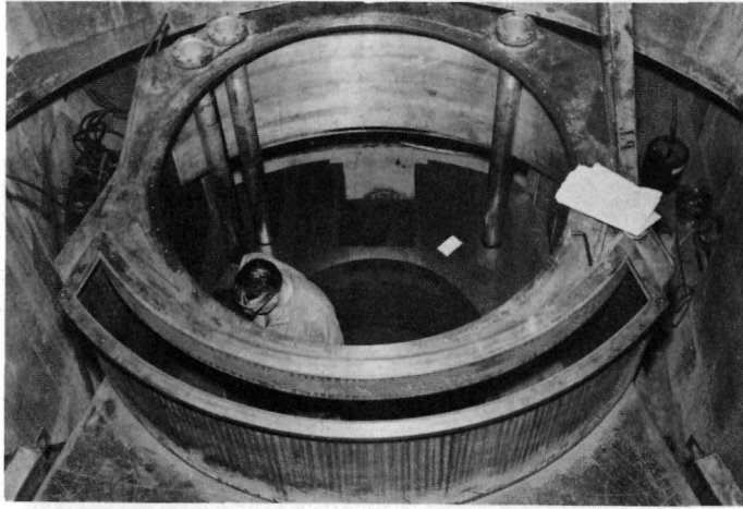
Fig. 33. Instrument Thimbles and Thermal-column Cavity Locations in Principal Graphite System
