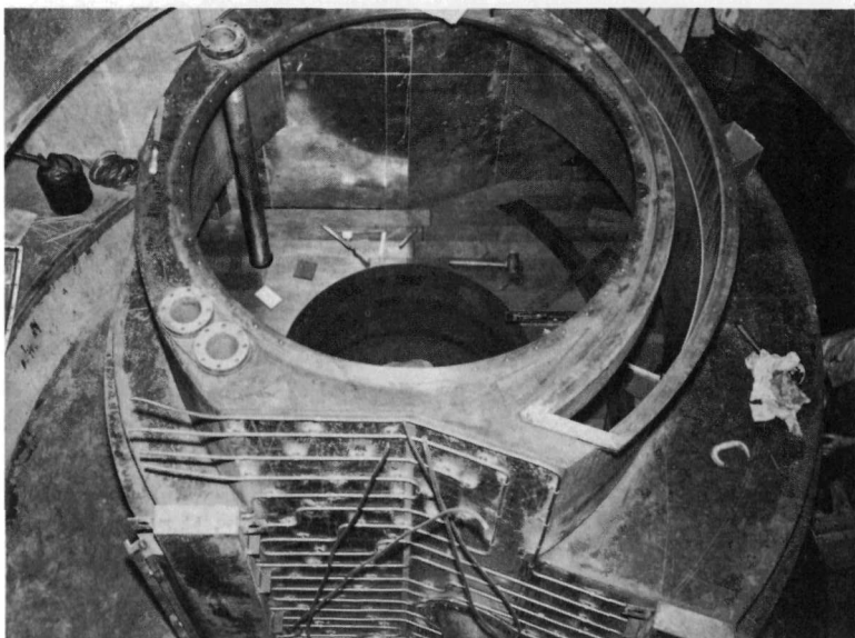
Fig. 8 Cooling Coils and Principal Graphite System Partly Installed
