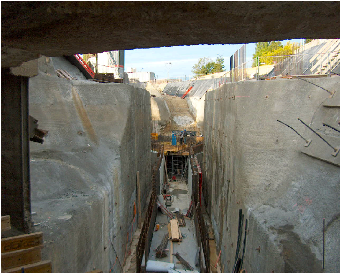
Fig. 6.7: Excavation of LINAC4 using the cut and cover technique.
