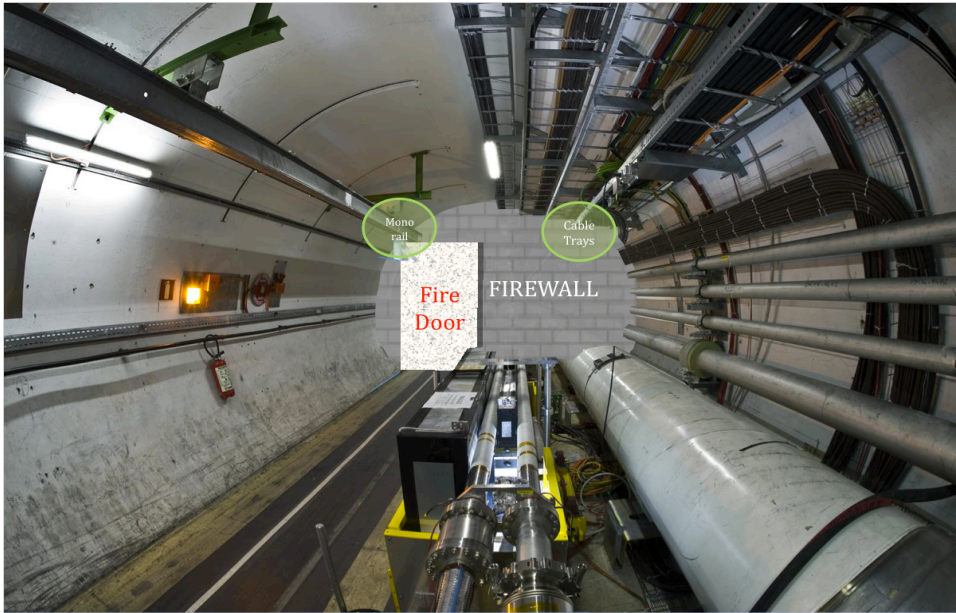
Fig. 6.37: Conceptual representation of a fire wall transversal to the tunnel orientation
