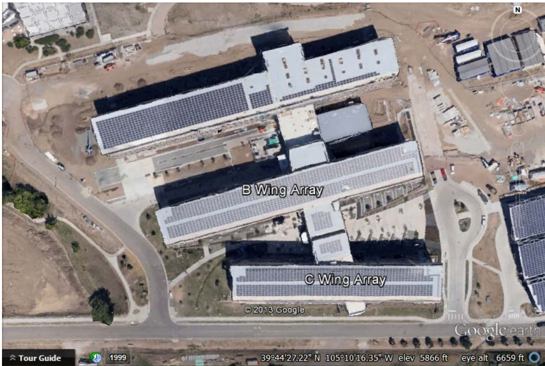
Figure 5-2. Aerial view of the RSF 1 system's BWA and CWA [10]
