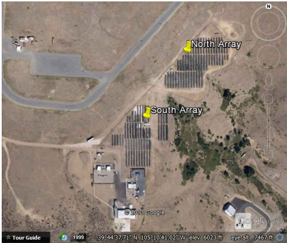
Figure 4-2. Aerial view of the Mesa Top system's north and south arrays [7]
