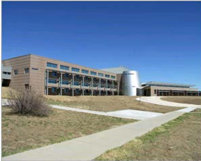
Figure 7-1. View of the S&TF [12]
