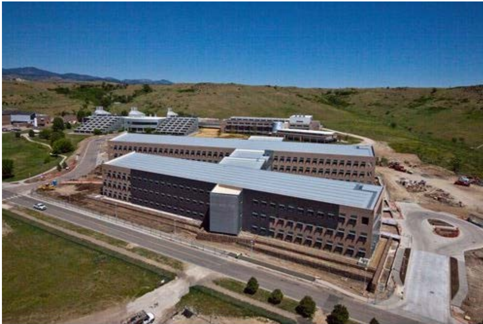
Figure 5-1. Aerial view of the RSF 1 system (picture 17767) [9]
