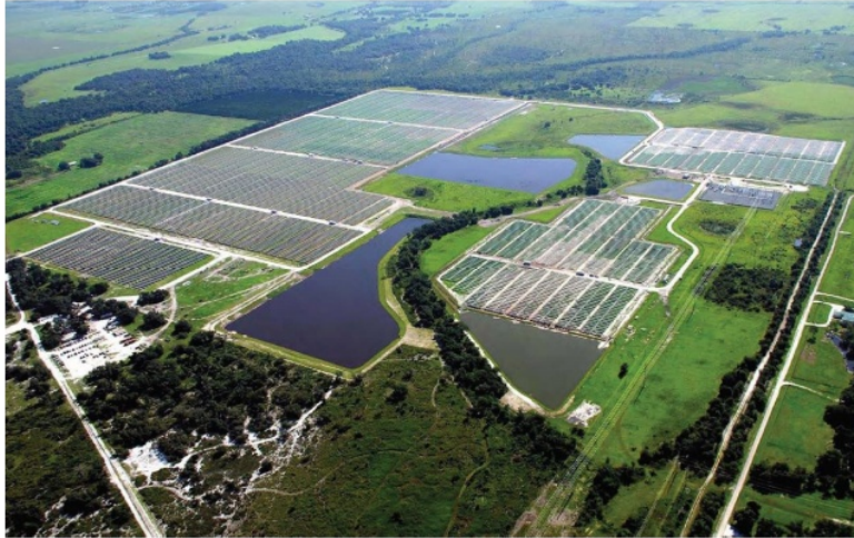
Figure 10-2. Aerial view of DeSoto [16]
