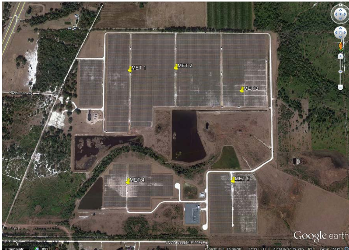
Figure 10-3. Five pyranometer locations near DeSoto [17]
