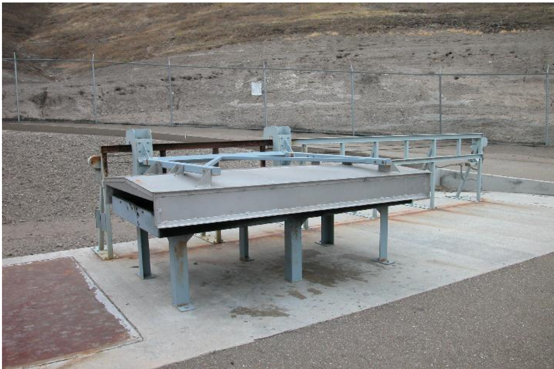
Figure 3. EWTF Burn Pan, covered.
