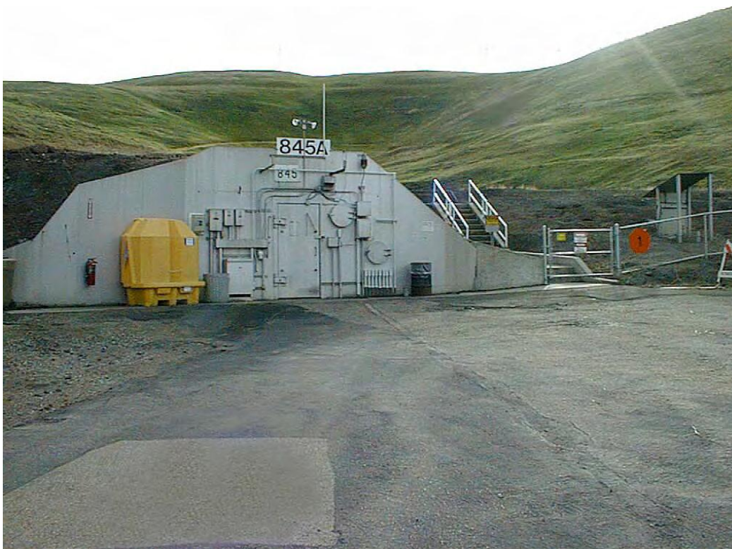
Figure 5. EWTF Control Bunker (Building 845A).
