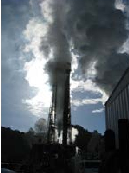
Figure 4: P-5 St-1 Flowing Steam While Installing Production Liner
