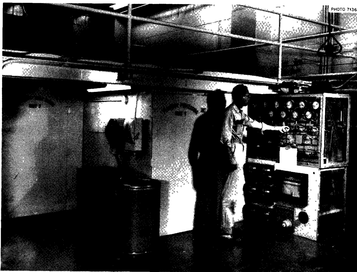
Fig. 16. Fluoride Production Facility – Process Control Unit.
