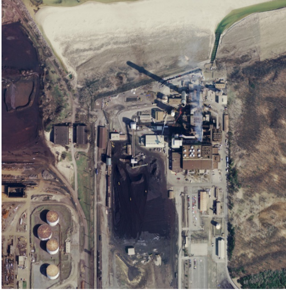
Figure 13. Coal-fired power plant, HP52.
