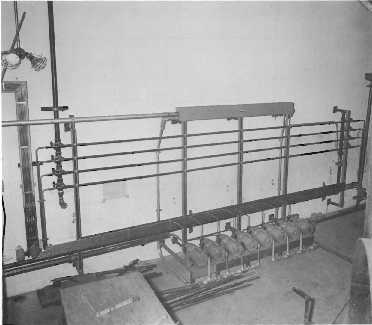
FIGURE 20. Pumps and Heat Exchangers for Liquid Sampling Loops
