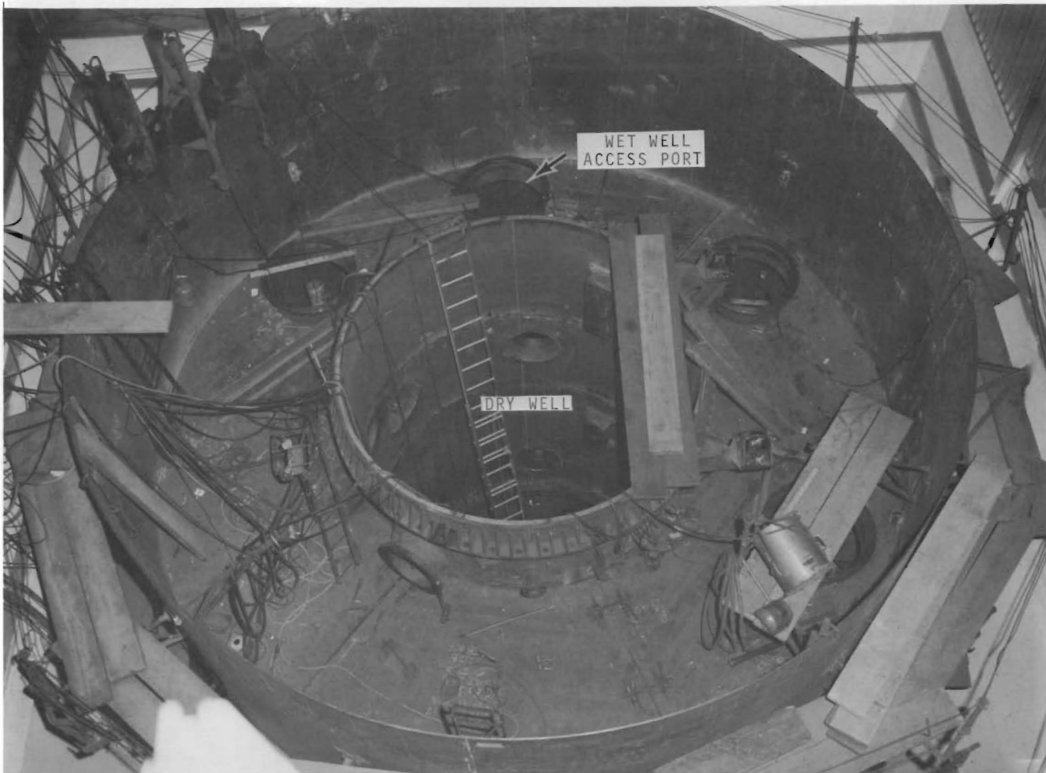
FIGURE 7. Interior View of Containment Vessel During Construction
