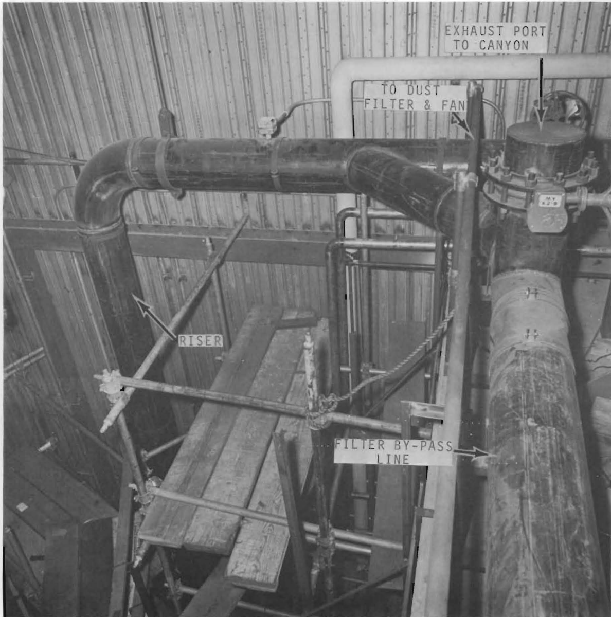
FIGURE 27. Exhaust Side of Ventilation Loop
