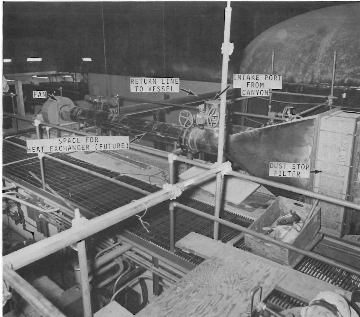
FIGURE 28. Dust Filter and Fan of Ventilation Loop
