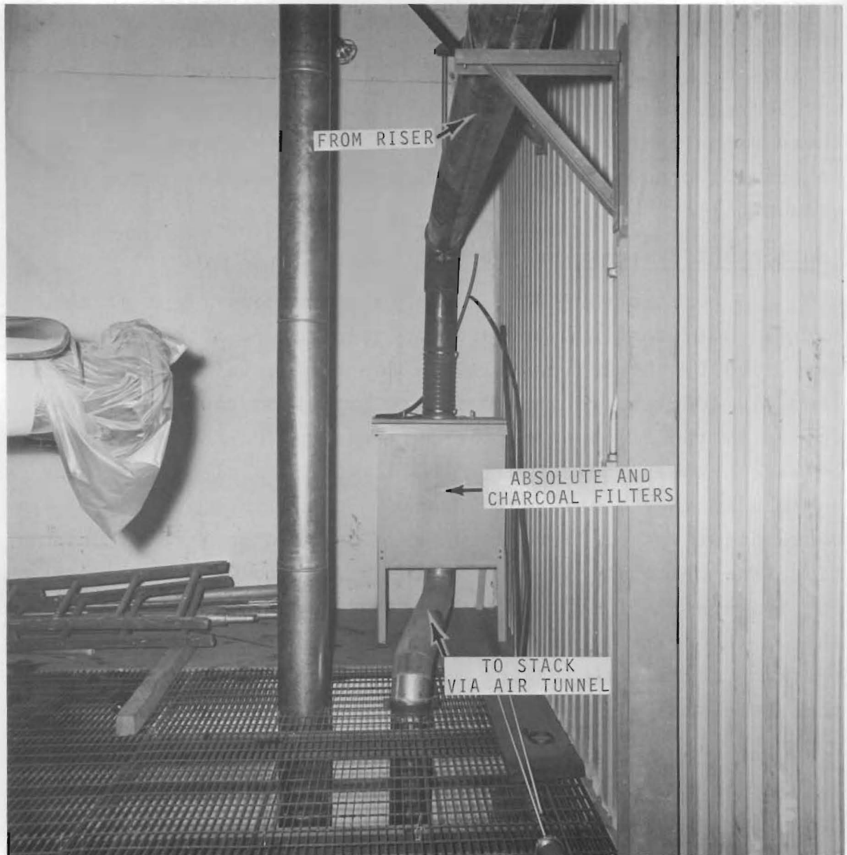
FIGURE 29. Line and Filter for Exhausting Contaminated Air
