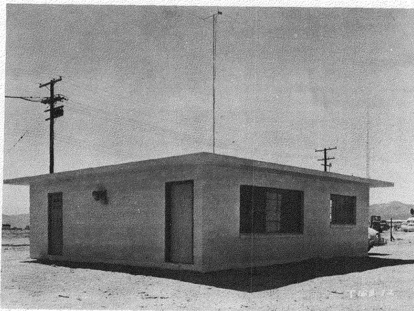
Fig. 2.18—One-story reinforced lightweight concrete-block house (31.1-f1) at 4700 ft, preshot.
