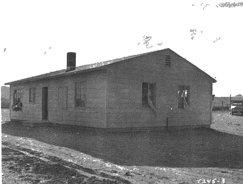
Fig. 3.54 —One-story frame rambler house (31.1-c2) at 10,500 ft, postshot.
