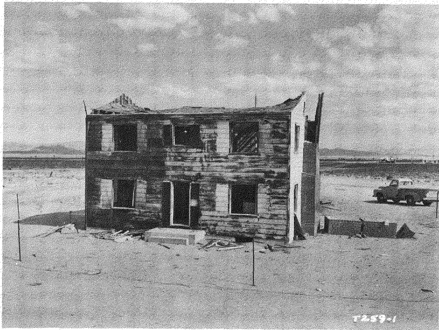
Fig. 3.21 — Two-story frame (strengthened) house (31.1-b1) at 5500 ft, postshot.
