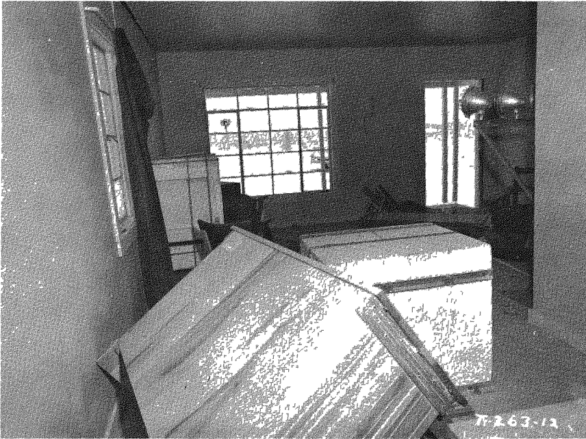
Fig. 3.51 —Interior of one-story reinforced lightweight concrete-block house (31.1-f2) at 10,500 ft, postshot.
