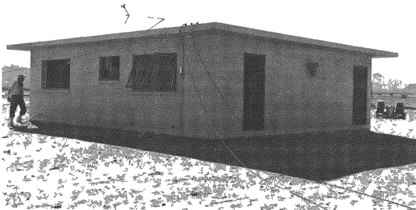
Fig. 3.18—One-story reinforced lightweight concrete-block house (31.1-f1) at 4700 ft, postshot.
