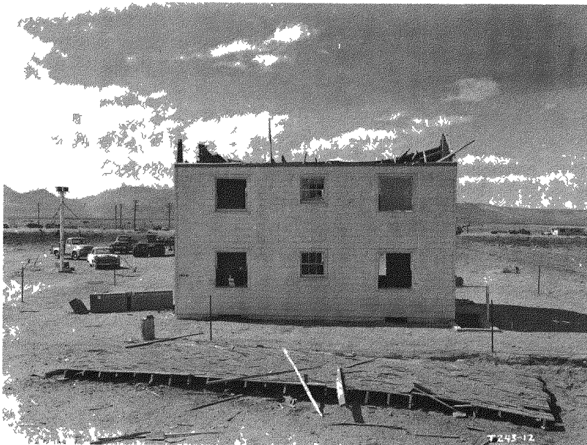
Fig. 3.24 —Two-story frame (strengthened) house (31.1-b1) at 5500 ft, postshot.
