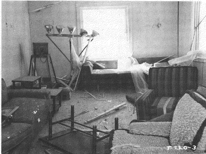
Fig. 3.34—Living room of the two-story frame house (31.1-b2) at 7800 ft, postshot.
