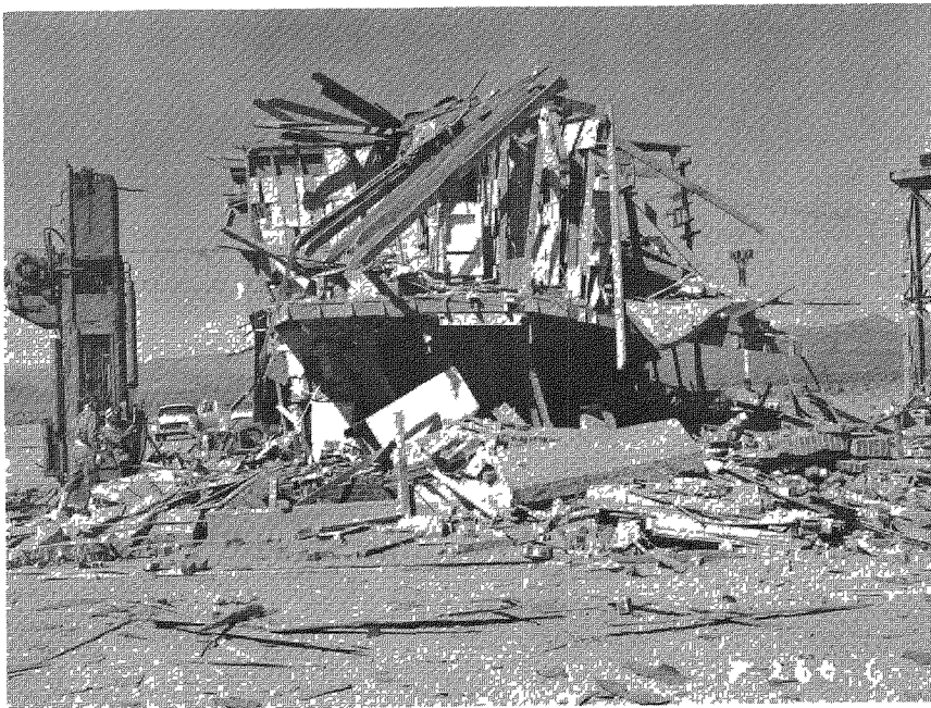
Fig. 3.4—Two-story brick house (31.1-a1) at 4700 ft, postshot.
