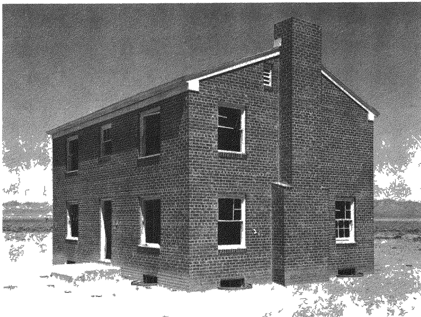
Fig. 3.42 —Two story brick house (31.1-a2) at 10,500 ft, postshot.
