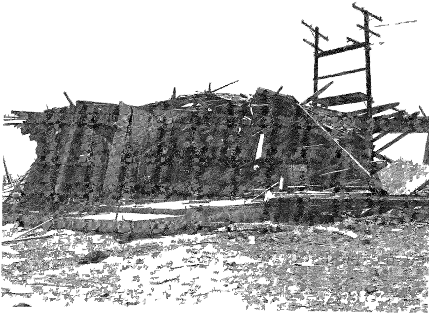
Fig. 3.6—One-story frame rambler house (31.1-c1) at 4700 ft, postshot.
