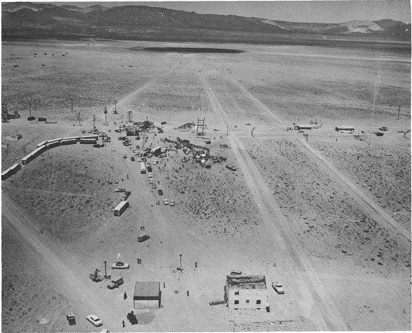
Fig. 3.2—Main FCDA test line, postshot, looking from middle distance toward GZ.
