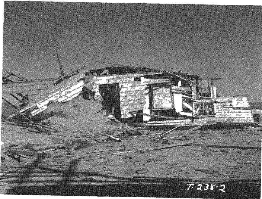
Fig. 3.7—One-story frame rambler house (31.1-c1) at 4700 ft, postshot, showing blast shutter and shelter undamaged.
