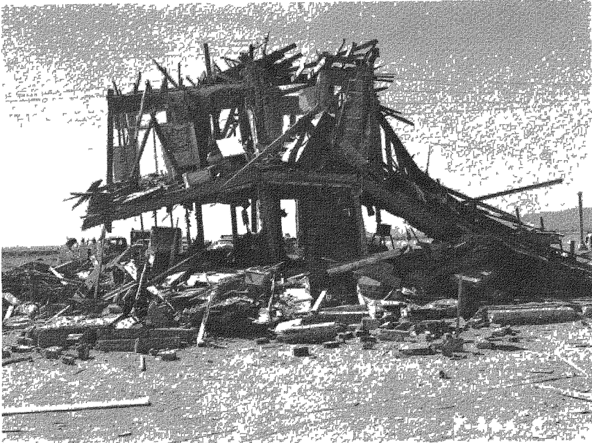
Fig. 3.3—Two-story brick house (31.1-a1) at 4700 ft, postshot.
