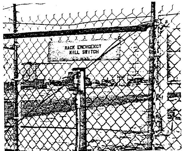
FIGURE 8-13. Emergency Loading Pump Stop Switch Located Remote From Rack at Property Entrance.
