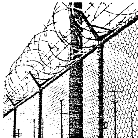
FIGURE 14-6. Double Bracket Mounting
