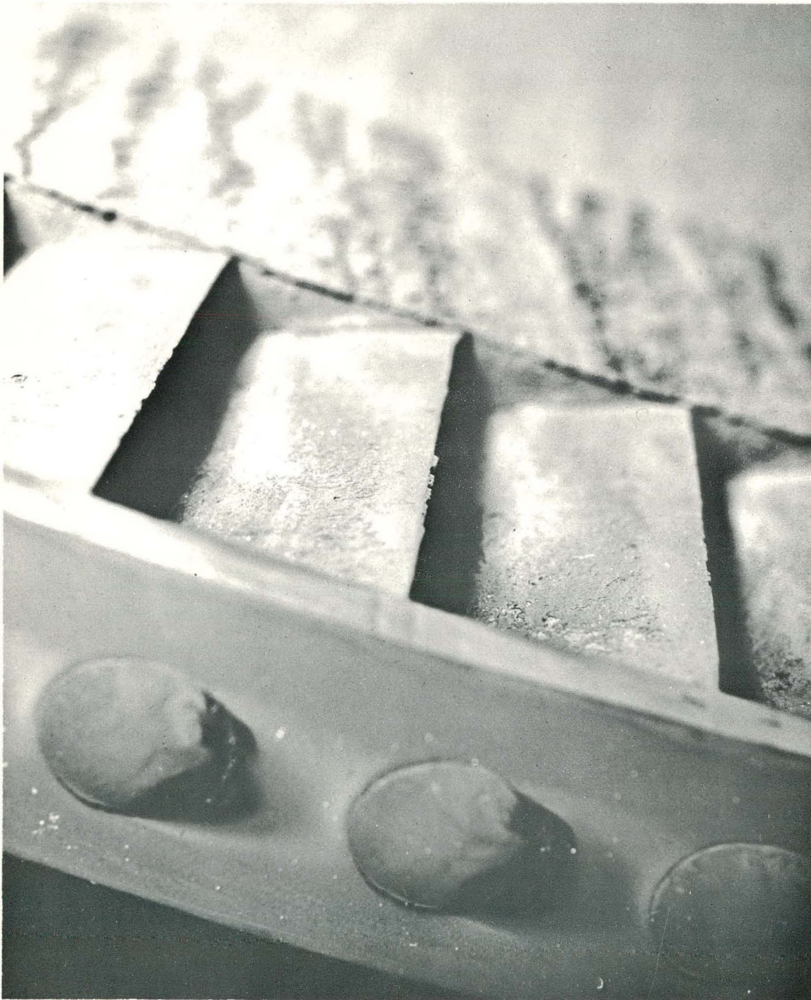
EXHAUST EDGE OF 2ND. CURTIS WHEEL BLADING
