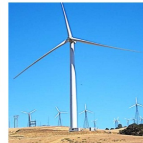
World's 1st GE 1.6-100 Hybrid powered by GE Durathon. Located at Tehachapi, CA
