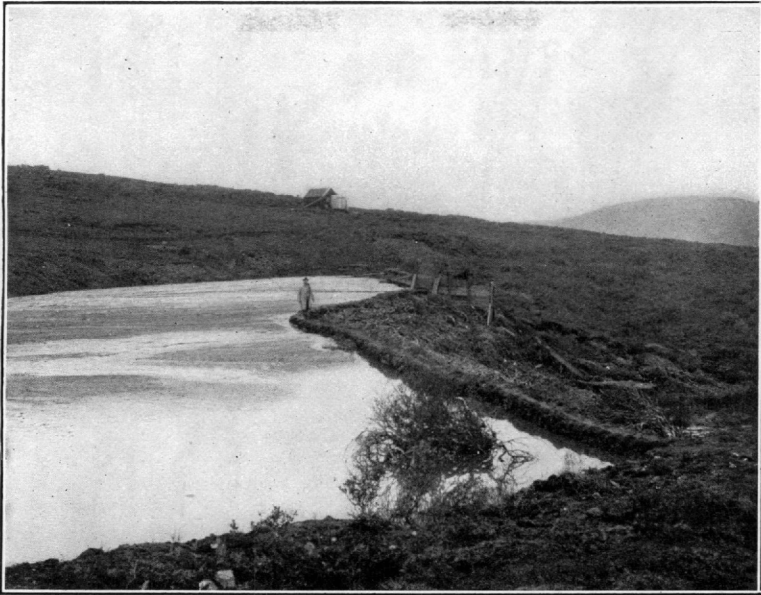
A. SETTLING POND, ANVIL CREEK, SEWARD PENINSULA.
