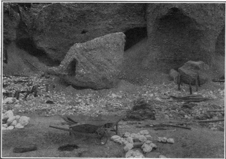
.II. BLOCKS OF FROZEN GRAVEL IN HYDRAULIC PIT, KLONDIKE.
