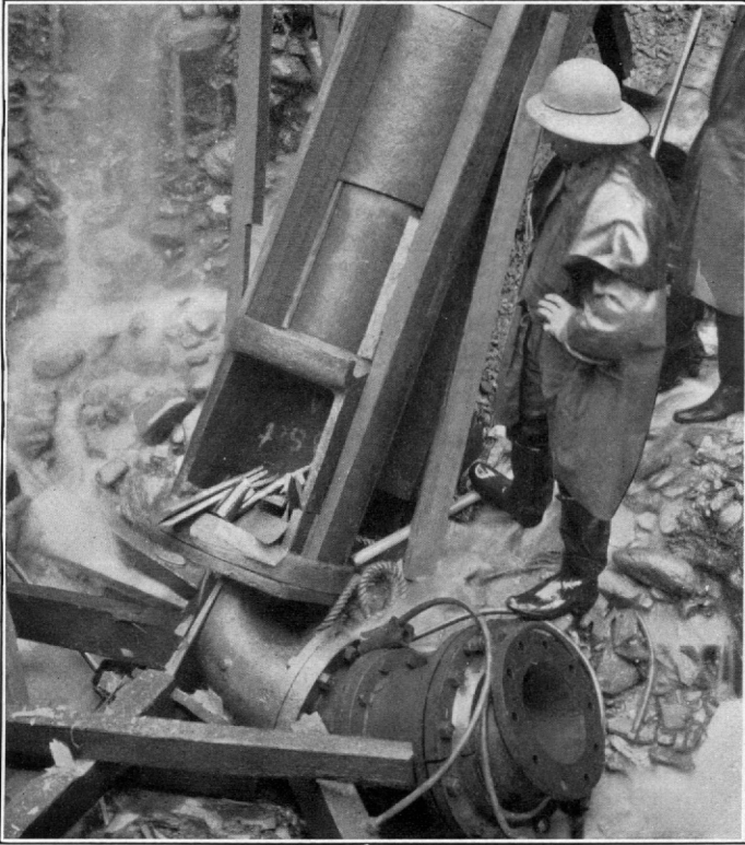
J. HYDRAULIC ELEVATOR IN PIT, GLACIER CREEK.
