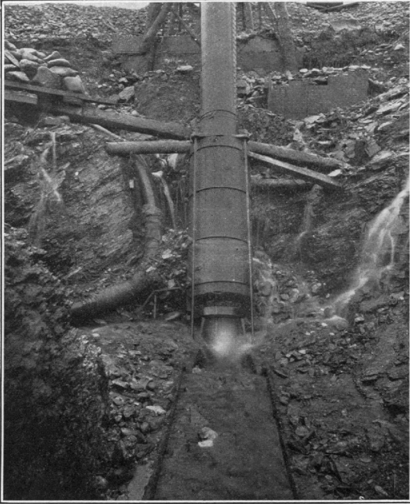
A. SLUICE BELOW ELEVATOR, OPHIR CREEK.
