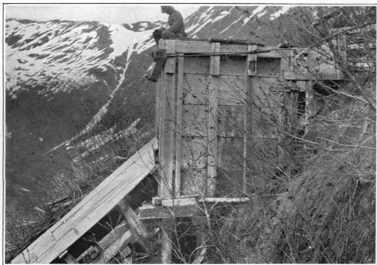
B. METHOD OF STAYING-PRESSURE BOX, SILVER BOW BASIN.
