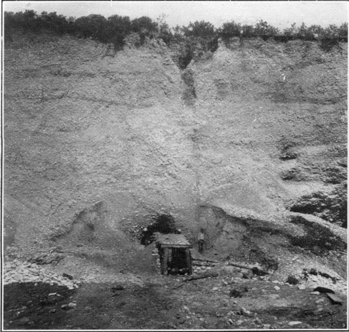
A. ADIT TO DRIFTING OPERATIONS.
