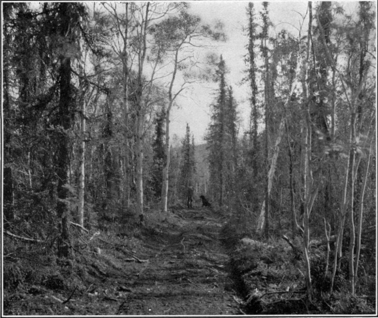
A. ROAD IN FAIRBANKS DISTRICT.
