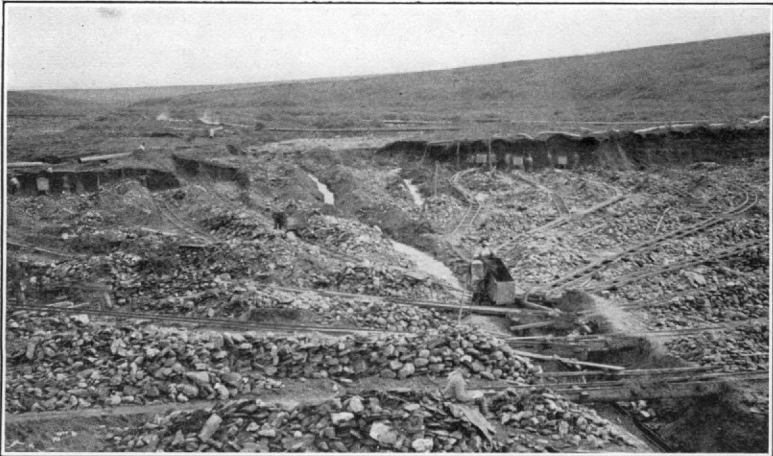
B. OPEN CUT WORKED BY TRAMMING TO BED-ROCK SLUICES.
