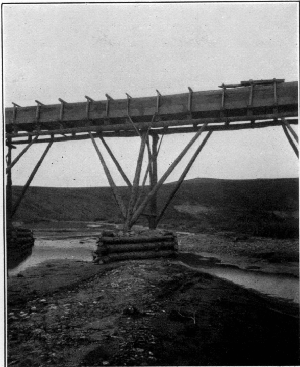
A. PIER FOR TRESTLE, HOT AIR DITCH LINE, OPHIR CREEK.
