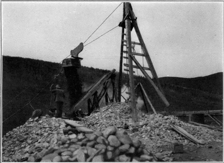
B. DUMPING TO SLUICES, KLONDIKE.
