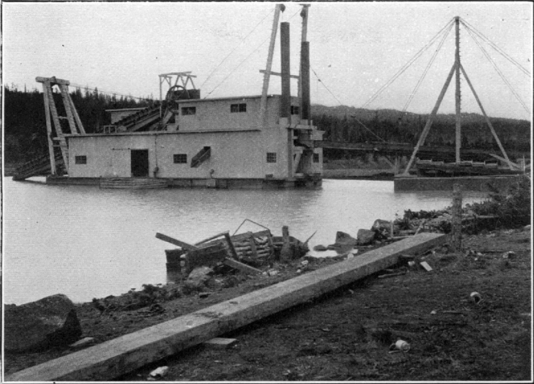
A. SINGLE-LIFT DREDGE, 40-FOOT GROUND AT ATLIN, COARSE GOLD.
