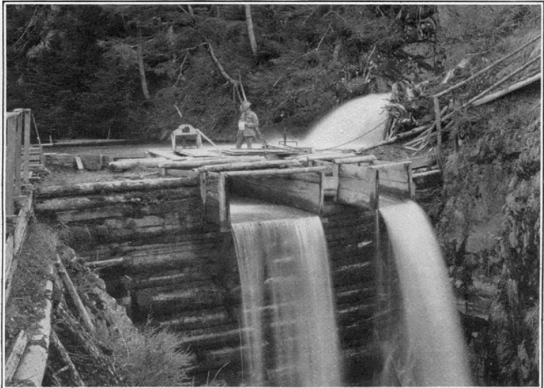
B. TREADWELL DITCH LINE AT LAWSON CREEK, DOUGLAS ISLAND.
