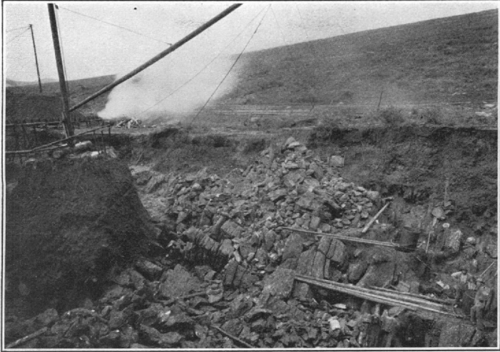
A. SKIDS FOR DERRICKING.
