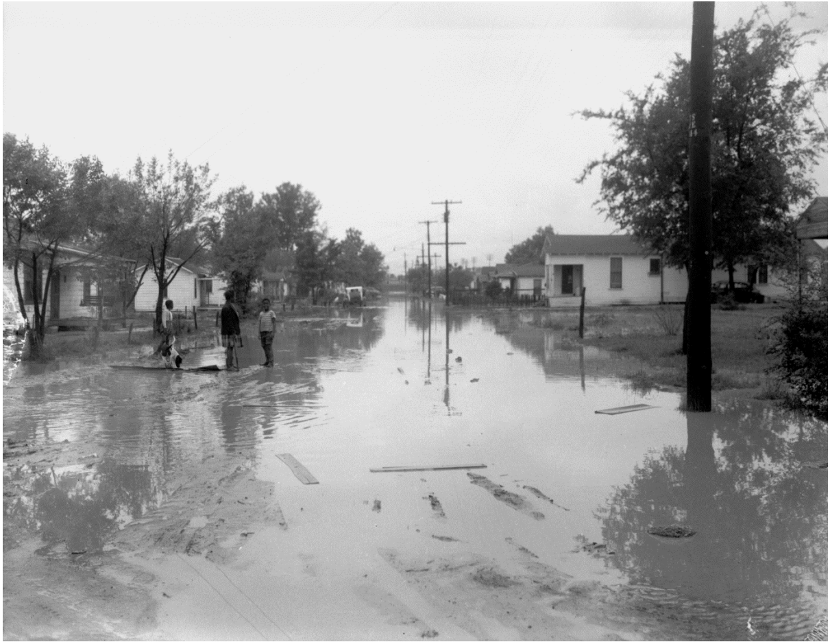
Figure 25: Flooding in the Bonton Addition of Dallas along St. Clara Street
