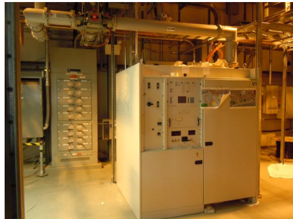
Figure 9: 500 MHz power amplifier for CeC PoP
