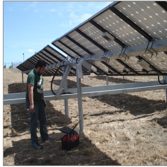
Figure 14. Installation of backside irradiance sensors on existing tracker system
