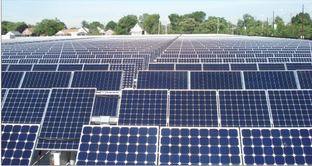
Figure 12: Bifacial modules interspersed with standard product commercial installation. Control (row 2) and bifacial modules (rows 3 and 4) field at commercial T0 site for continuous string monitoring
