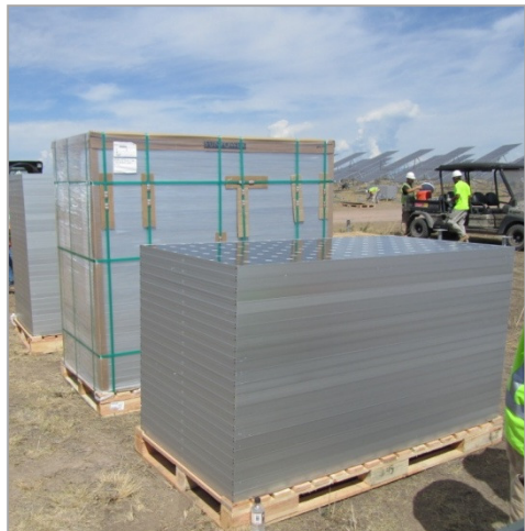
Figure 20: SunPower's 128-cell modules shown (i) palletized on job site and (ii) during installation on T20 v2.3 tracker
