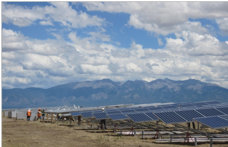
Figure 20: SunPower's 128-cell modules shown (i) palletized on job site and (ii) during installation on T20 v2.3 tracker
