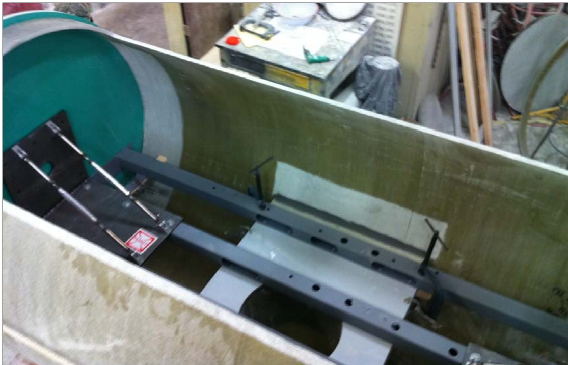
Figure 7 - Main structural frame rail installation into nacelle.
