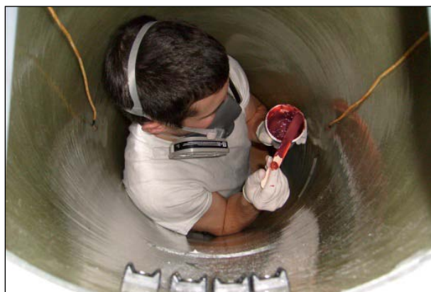
Figure 32. Sealing and waterproofing of structural strain gauges.
