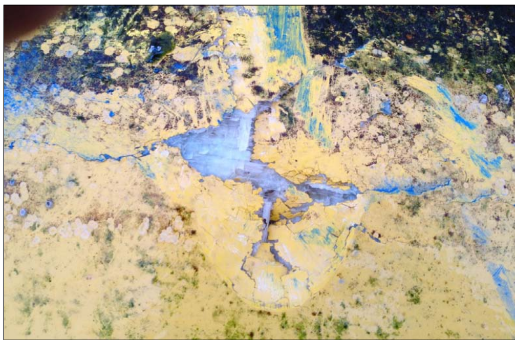
Figure 41 - Collision damage to the aft float FRP structure.
