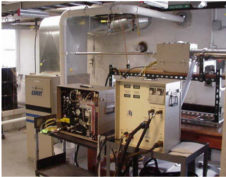
Figure 10. Oil-fired condensing warm air furnace, 95% AFUE rating
