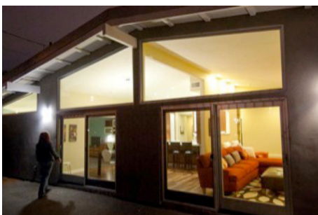
This 1963 Las Vegas home got new insulation, windows, and a new roof to cut energy use by 60%.
