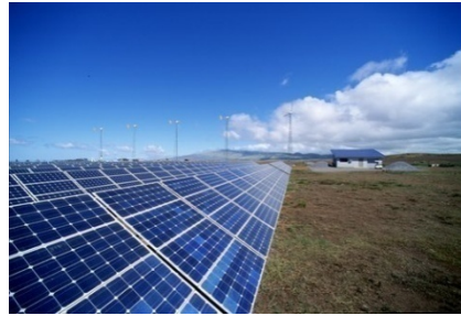
Source: NREL PIX 13823
