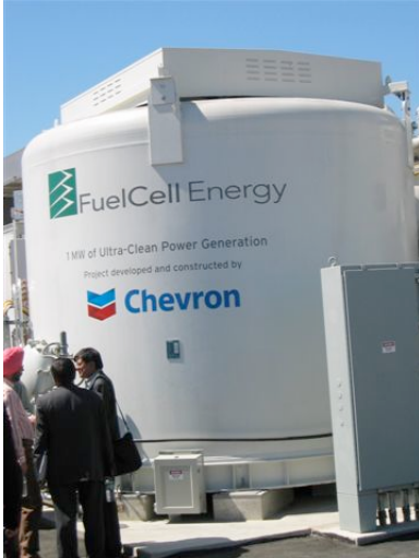
Fig. 2. The 1 MW Fuel Cell at Santa Rita Jail The fuel cell at the jail was intended to provide a consistent base load of 1 MW. The fuel cell’s performance has not been good. In fact, it produced at a 100% capacity factor in only one month over the 2007-2009 period. The missed 2009 bill savings resulting from less-than-perfect performance are shown in Figure 3.
