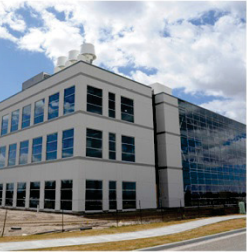
The Research Education Laboratory (REL) , slated for completion in 2014, will be the research and development and National Scientific User Facility high-performance gateway to INL, supporting nuclear fuel cycle research, site stewardship, research involving industrial processes, and advanced energy generation.
