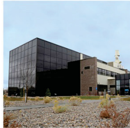
The Energy Systems Laboratory (ESL) , dedicated in April 2013, provides support infrastructure to enhance the nation's global competitiveness by advancing energy security through integration of clean energy systems, advancement of energy storage technologies, and biomass design and analysis.
