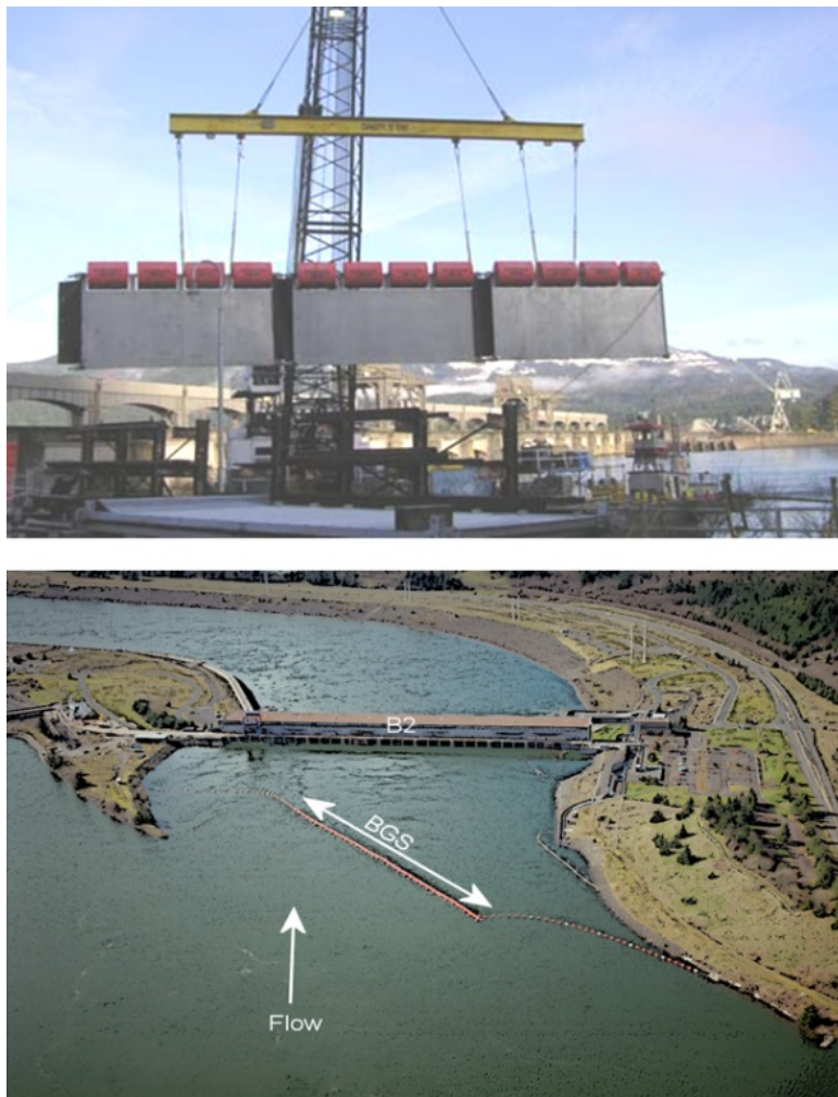
Figure 1.2. The Behavioral Guidance Structure with One Section Shown out of the Water (top); and as Deployed in the Forebay of the Bonneville Dam Second Powerhouse (B2; bottom)
