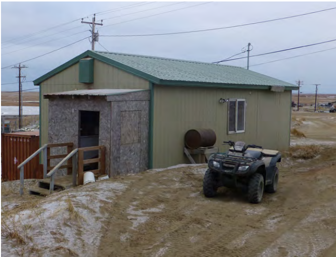
The Blaze Tinker House. Arctic Entry constructed by resident.
