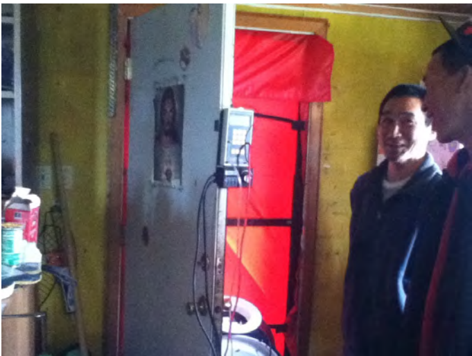
Local trainees received training in performing a blower door test. Eric Whitney of Bethel was the instructor.
