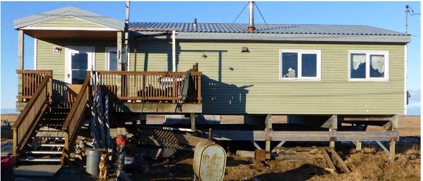
Moses Night House. Exterior view.
