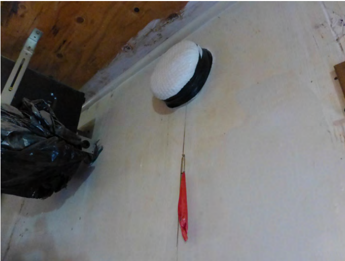
Ventilation system from a prior weatherization attempt has been disabled.
