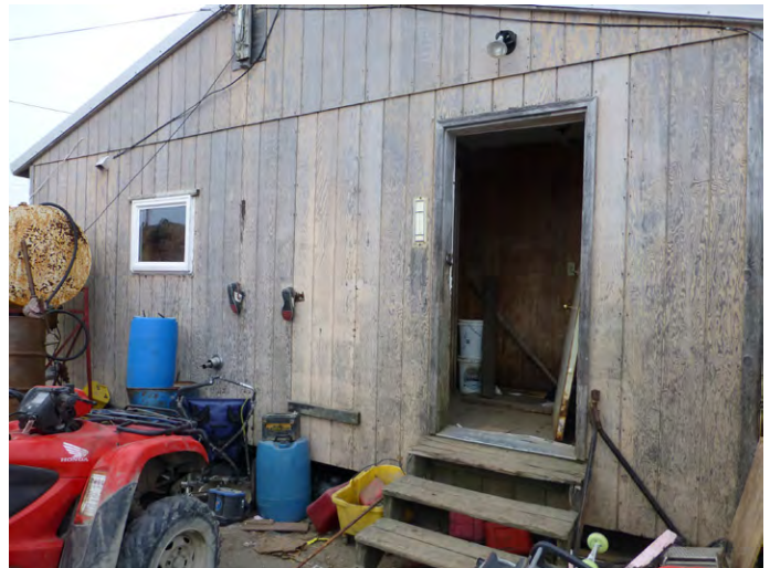
Leonard Bell House. The home has an interior arctic entry.
