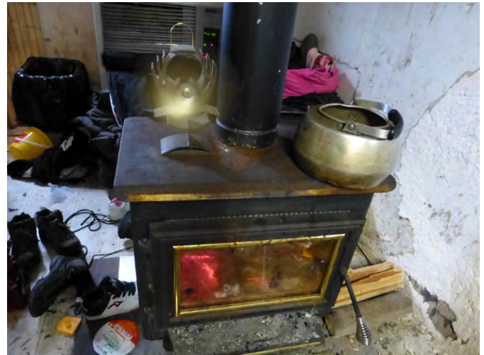
A passive fan atop the woodstove moves heat laterally into the living area.
