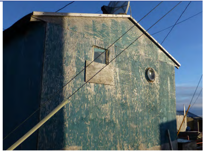
Henrietta Naneng House. Exterior view.
