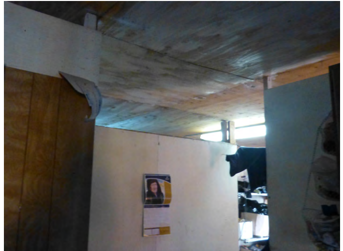
Interior walls are cut short of floor and ceilings to allow heat to move from room to room.
