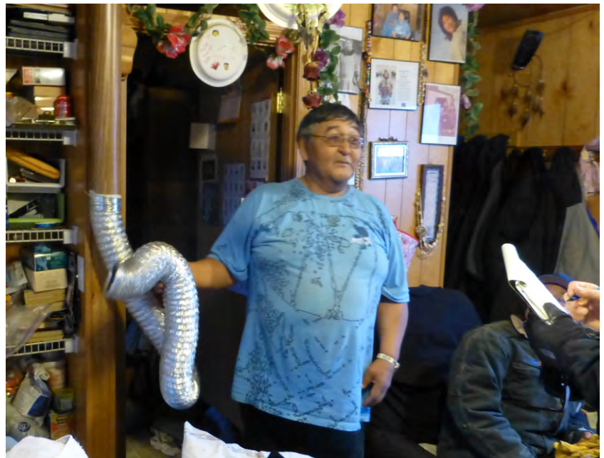
Harvey and Mary Tinker House. The resident has constructed a passive air exit vent that can be moved to the floor or higher in the home during the winter and summer, respectively. The intake air is through a Fresh 80 vent.
