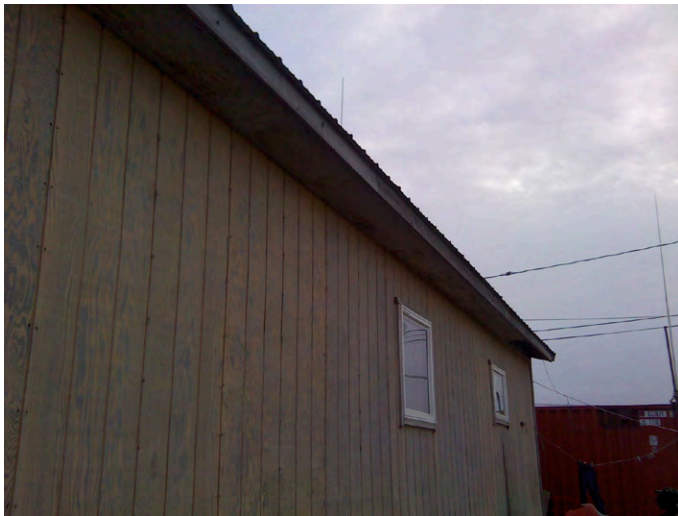
Leonard Bell House. View of eaves.
