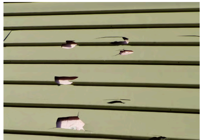
Moses Night House. Exterior rigid insulation was applied during a prior retrofit.
