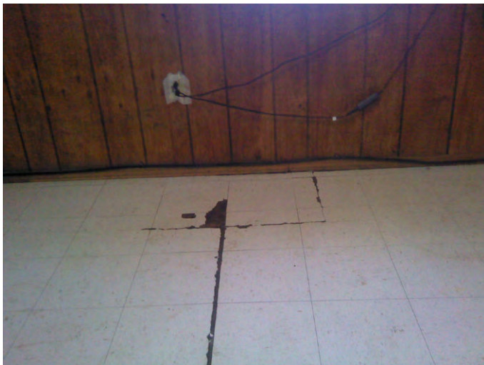
Leonard Bell House. View of floor where it meets an exterior wall
