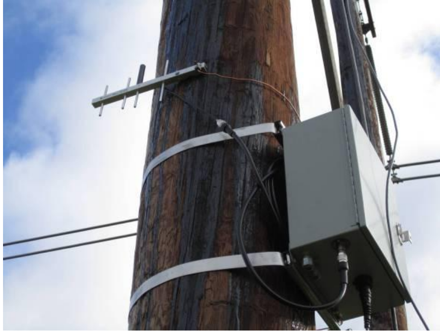
Figure C-34 ThermalRate electronics box and antenna
