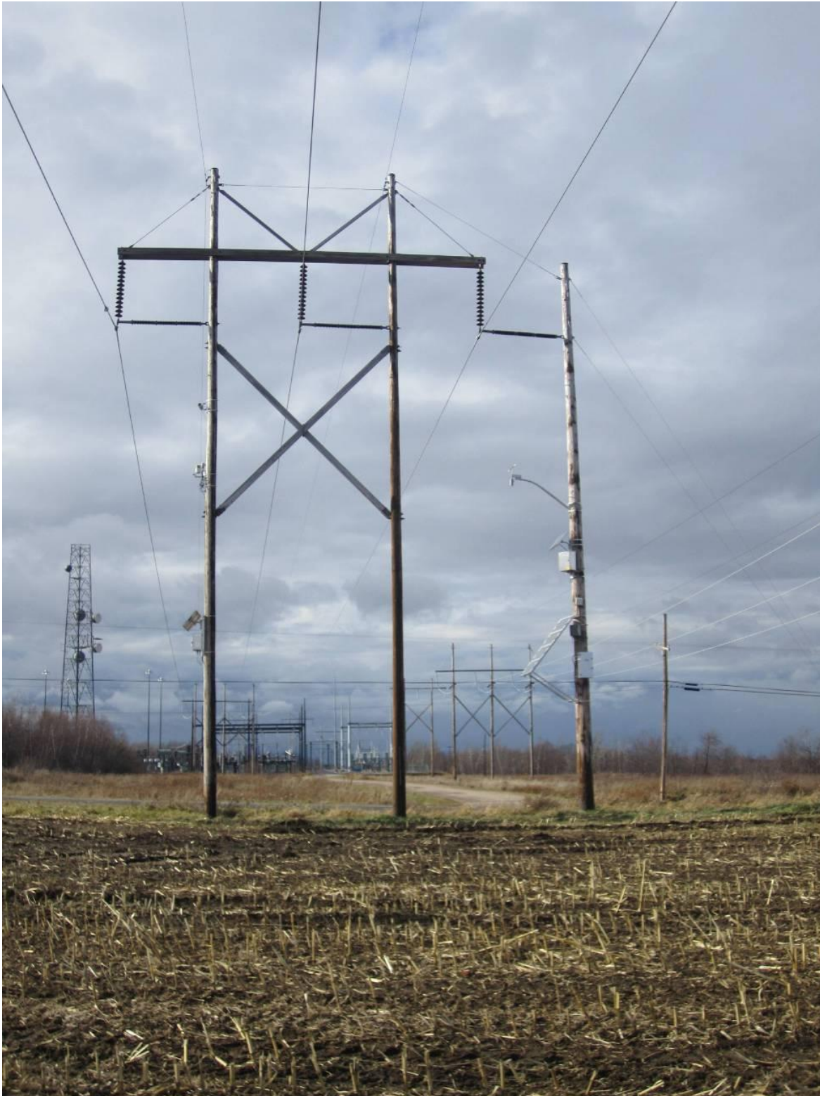
Figure C-52 Site 1 Completed – Looking in a Westerly Direction
