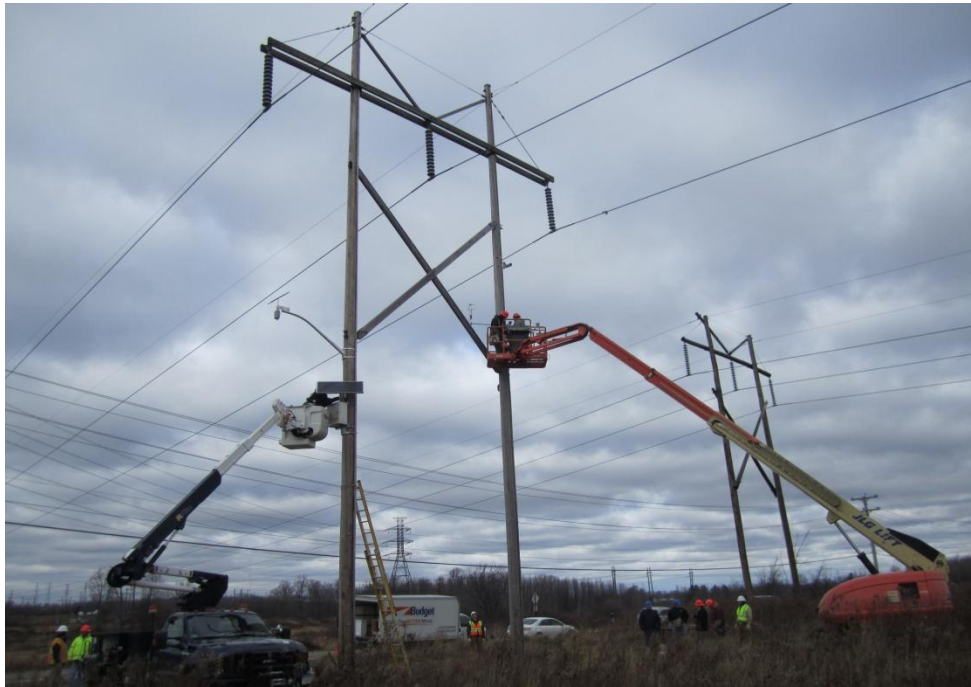
Figure 6-1 Installation of equipment on a NYPA line
