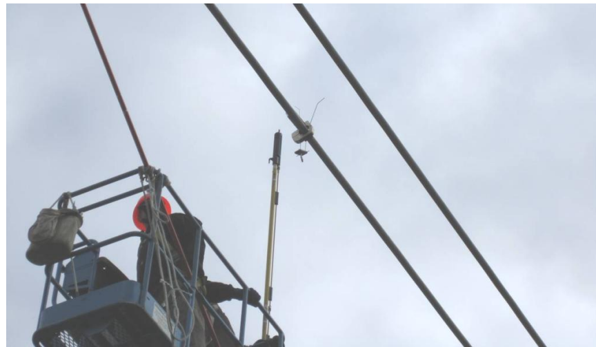
Figure C-31 Bonding tip becomes stuck during the first install attempt
