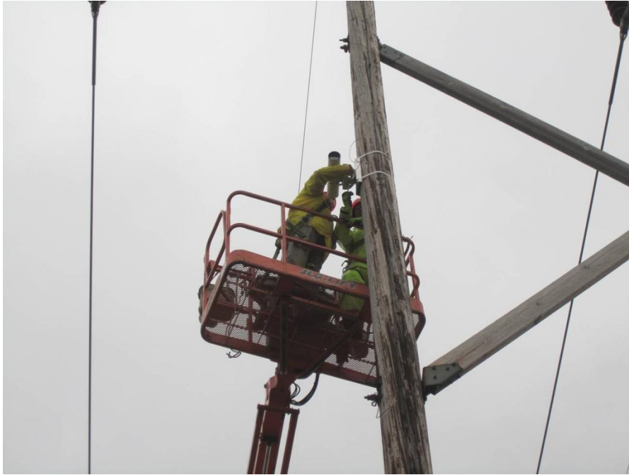
Figure C-60 Installed the Sagometer Camera
