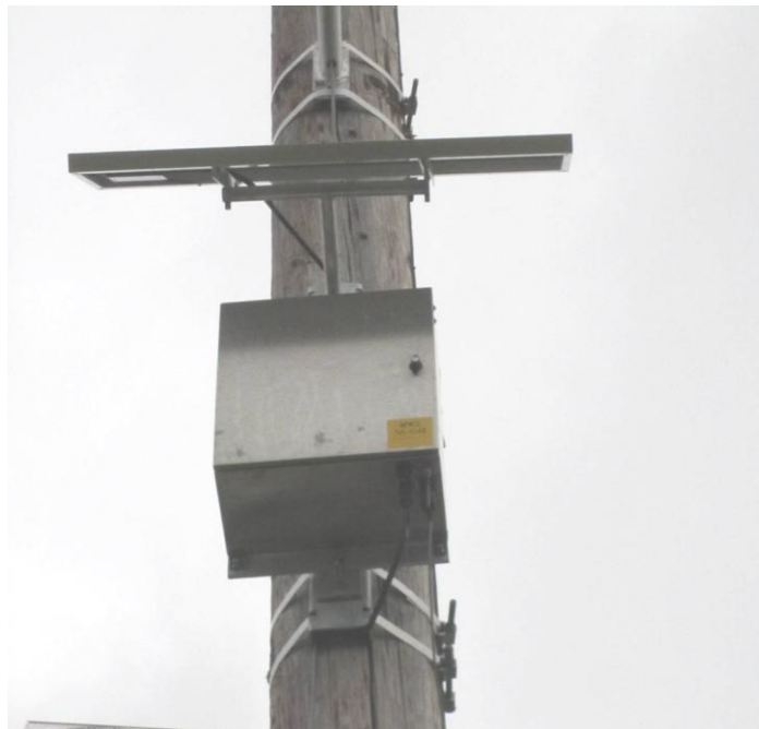
Figure C-54 EPRI Sensor Electronics Box and Solar Panel Installed
