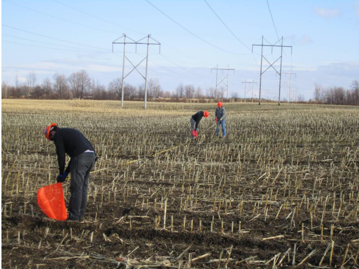
Figure C-39 Locations were marked under the line for the sagometer target and EPRI sensors.
