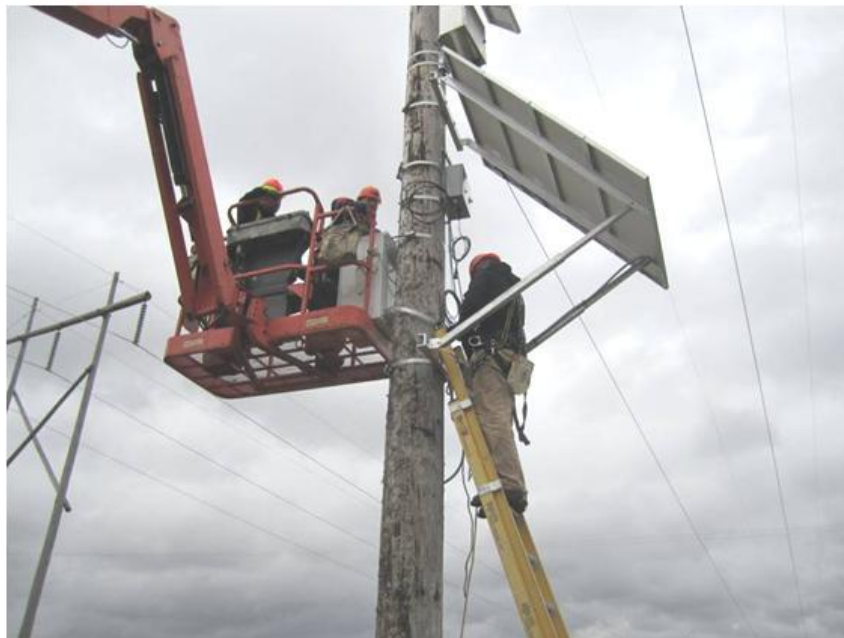
Figure C-58 ThermalRate System Solar Panel and Electrical Box Being Installed
