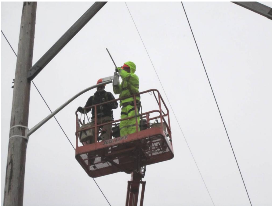
Figure C-57 Installing the ThermalRate Sensor
