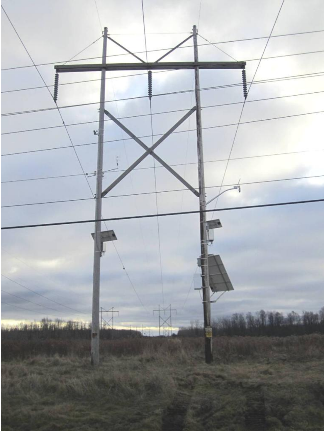
Figure C-74 Site 3 Completed – Looking Back in the Direction of Willis Substation
