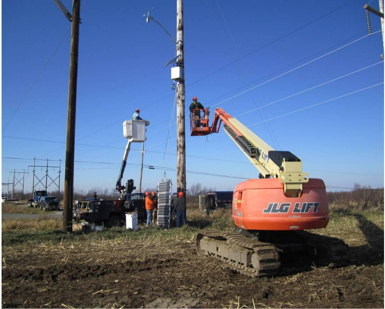
Figure C-46 Solar panel for the ThermalRate system being rigged for installation
