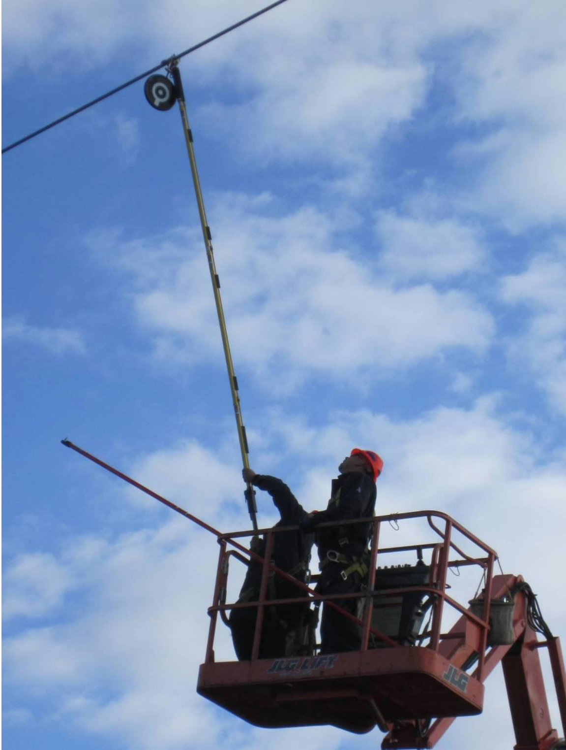
Figure C-49 Sagometer Target Being Installed
