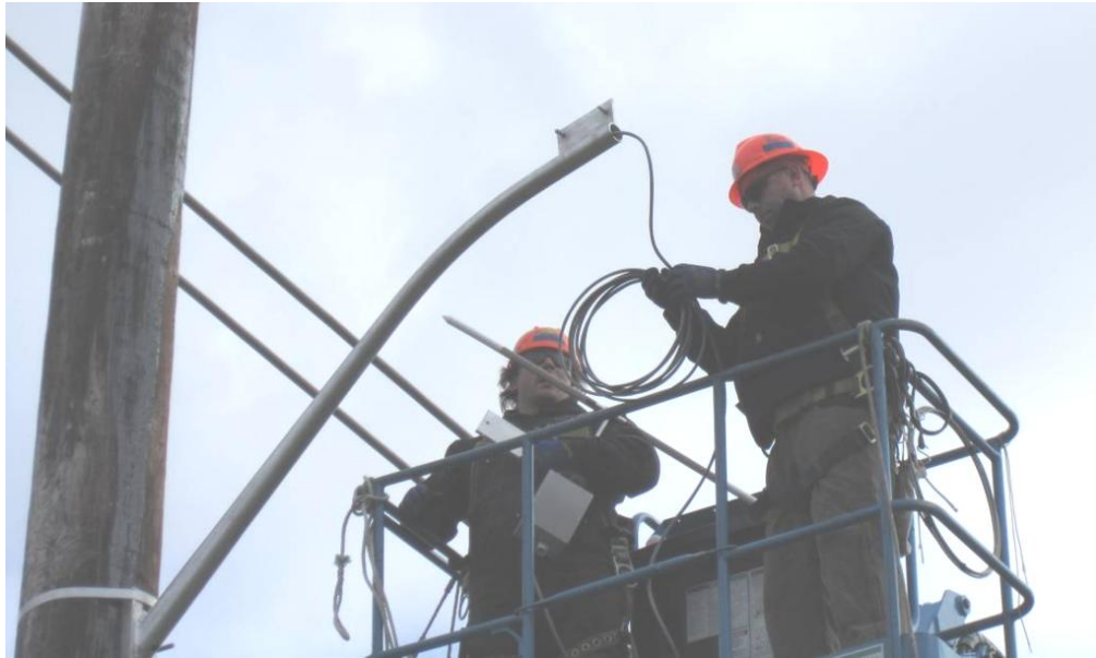
Figure C-32 ThermalRate sensor being prepared for mounting
