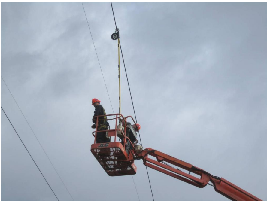
Figure C-61 Installing the Sagometer Target
