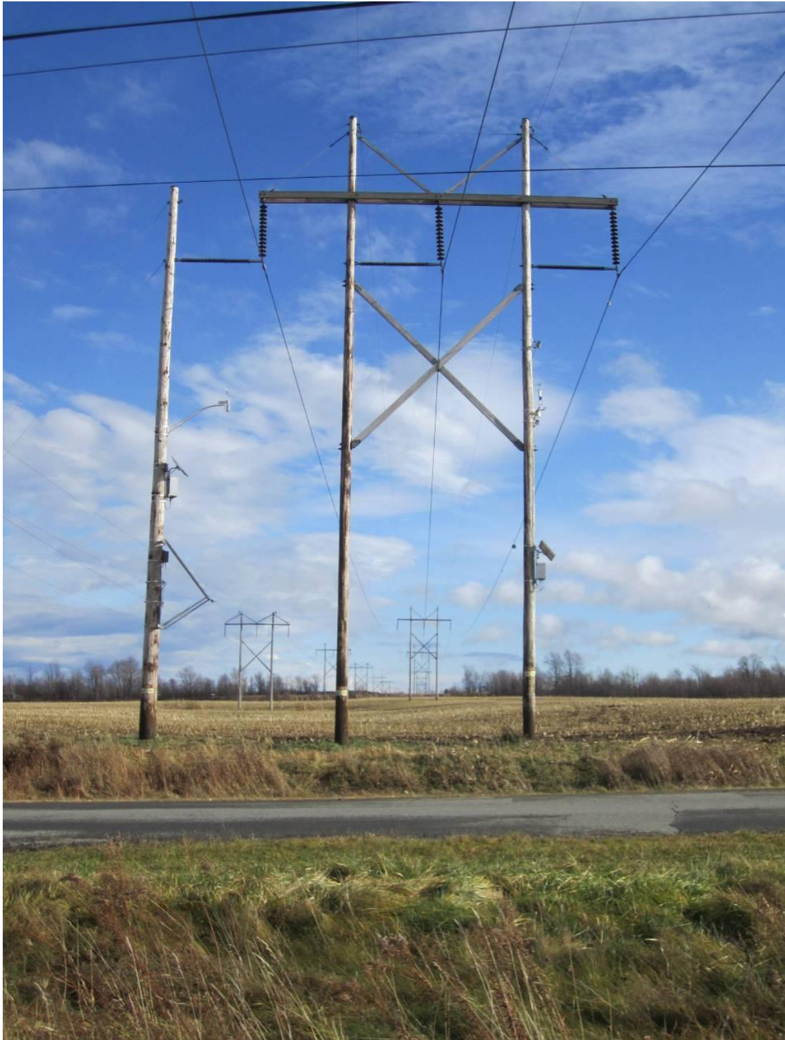
Figure C-51 Site 1 Completed – Looking in an Easterly Direction
