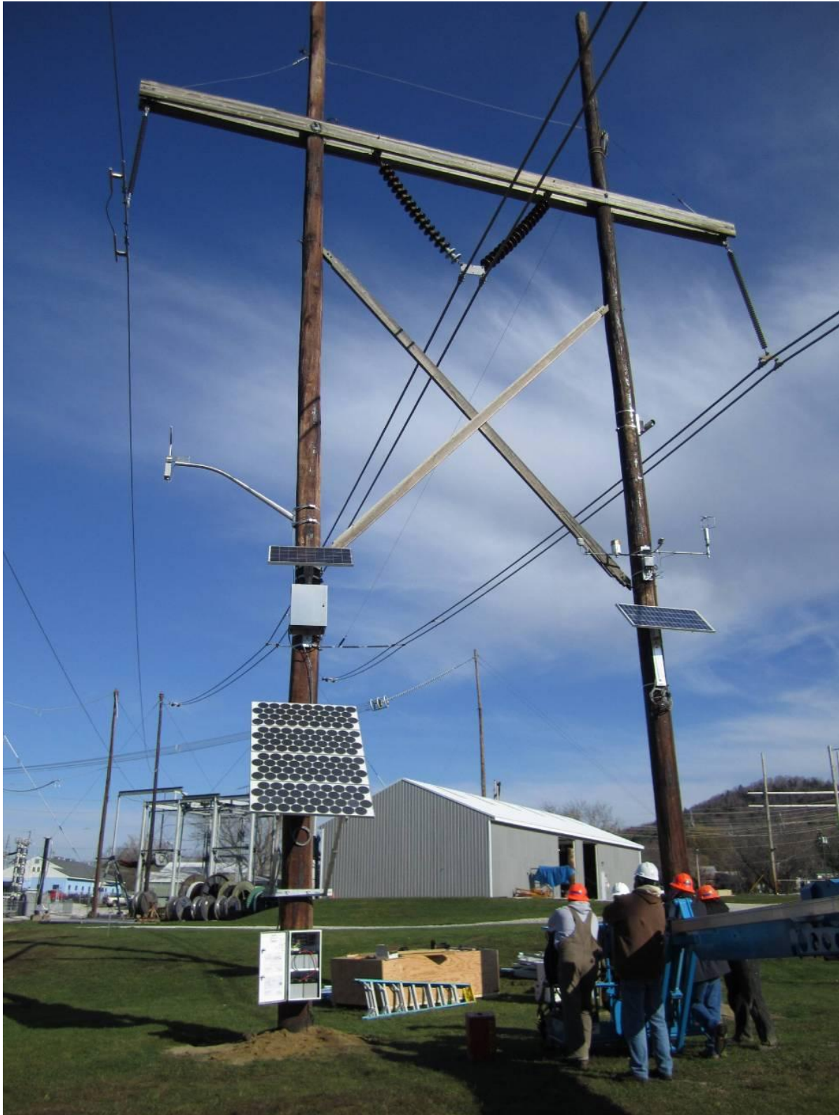
Figure C-38 Near completion of the practice installation at EPRI Lenox
