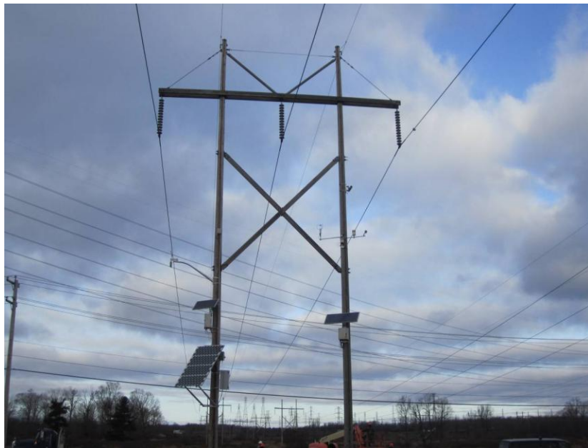
Figure C-73 Site 3 Completed – Looking Toward the Substation
