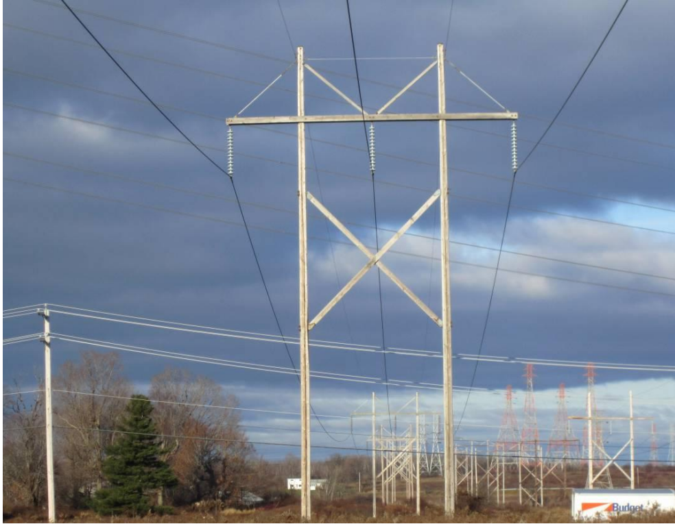
Figure C-72 Looking Back at Structure Site 3 Before Installation Begins
