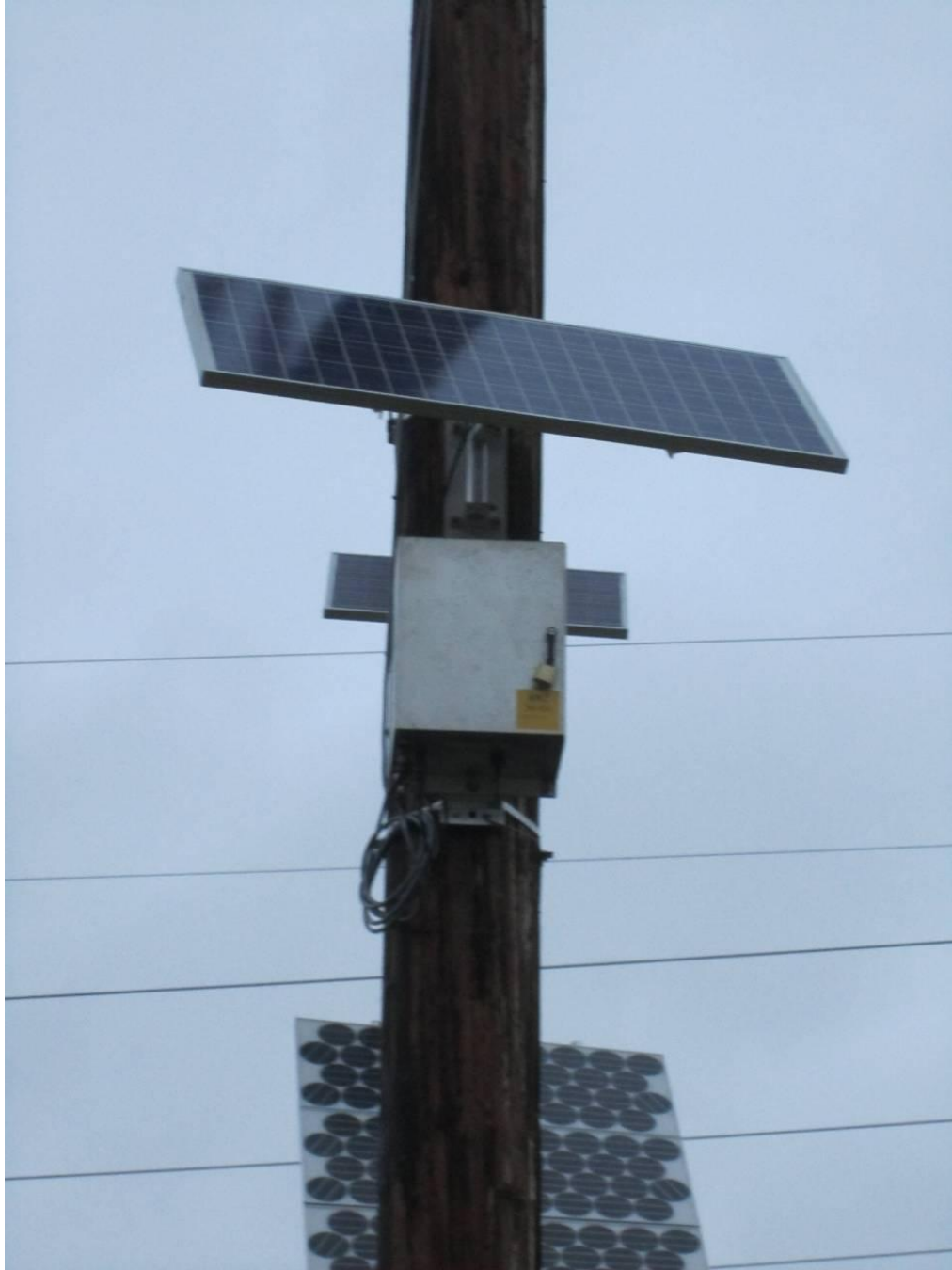
Figure C-63 Sagometer Electronics Box and Solar Panel Installed
