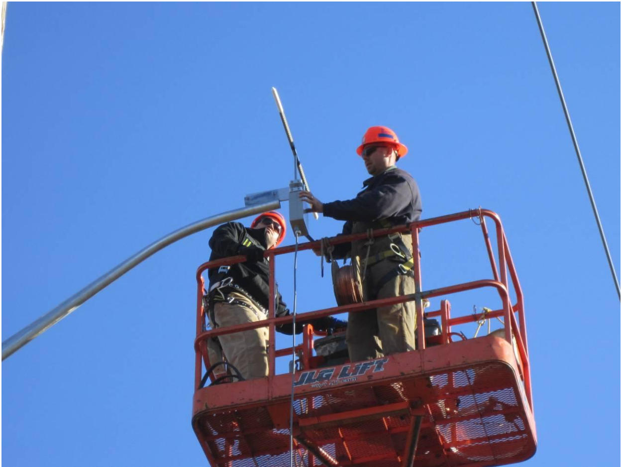
Figure C-45 ThermalRate sensor being installed
