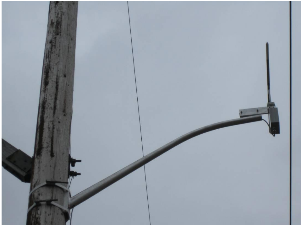
Figure C-67 ThermalRate Sensor and Arm Installed
