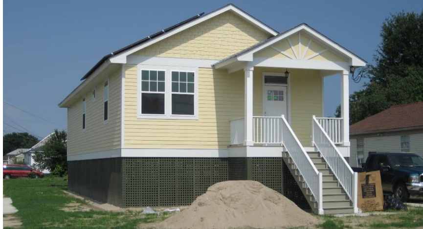
Figure 6. Phase VI house under construction
