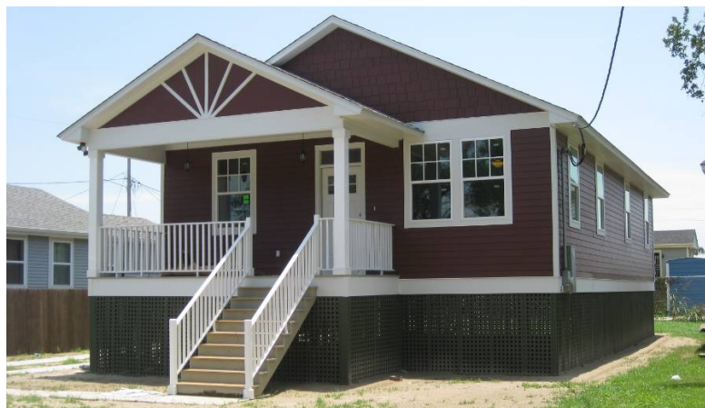
Figure 3. Phase V house under construction
