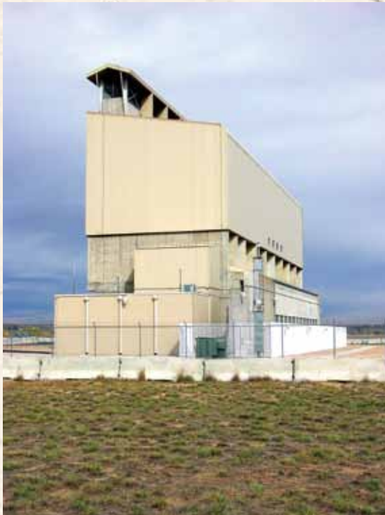
Fort St. Vrain Modular Vault Dry Store
