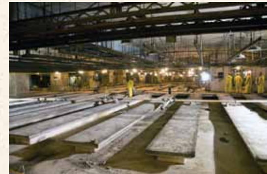
Grouting of Savannah River Site R Reactor Disassembly Basin.
