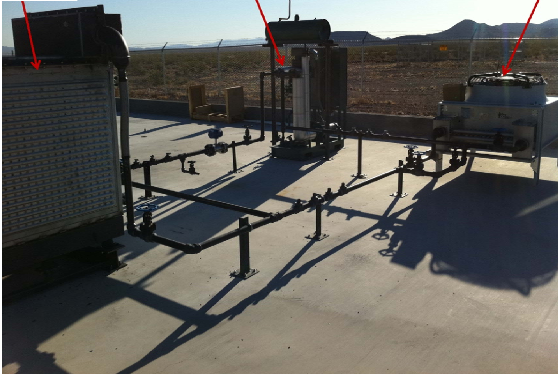
Figure 8 – Test loop equipment anchored with piping, valves, and instrument wells installed.
