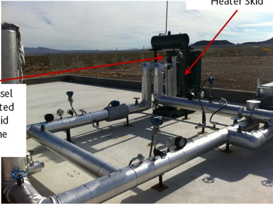
Figure 23 – Expansion vessel elevation before test loop modifications.
