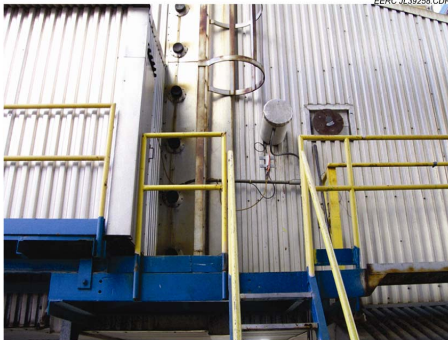
Figure 6. Port locations for sampling. Rightmost port was location for mercury CEM.
