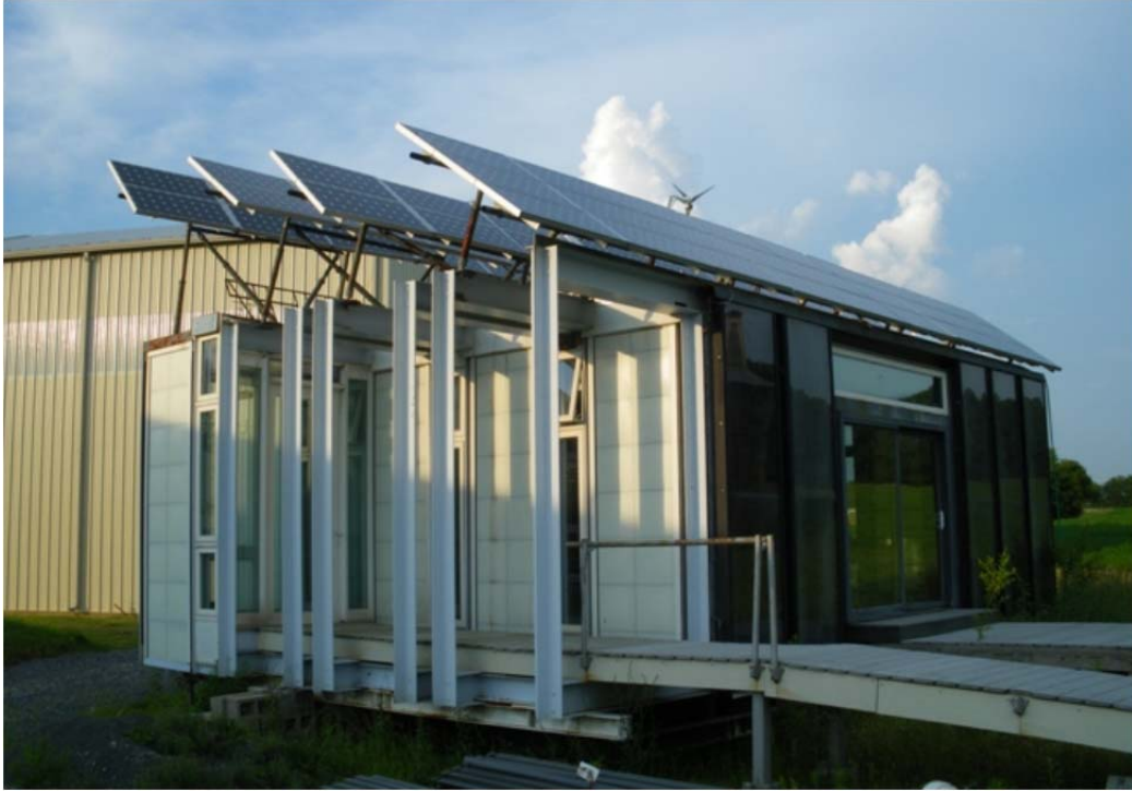
Figure 2.3. Photograph of VT solar house for power conditioner energy production study.
