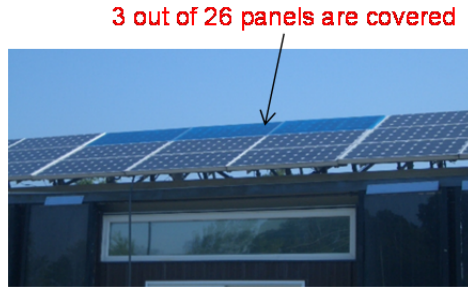
Figure 2.11. Photograph showing manually created partial shading for the three PCS groups.
