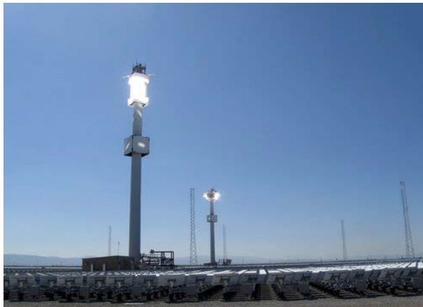
Figure 7.1-5 eSolar's Sierra SunTower Facility outside of Lancaster, California (NREL 2010b)
