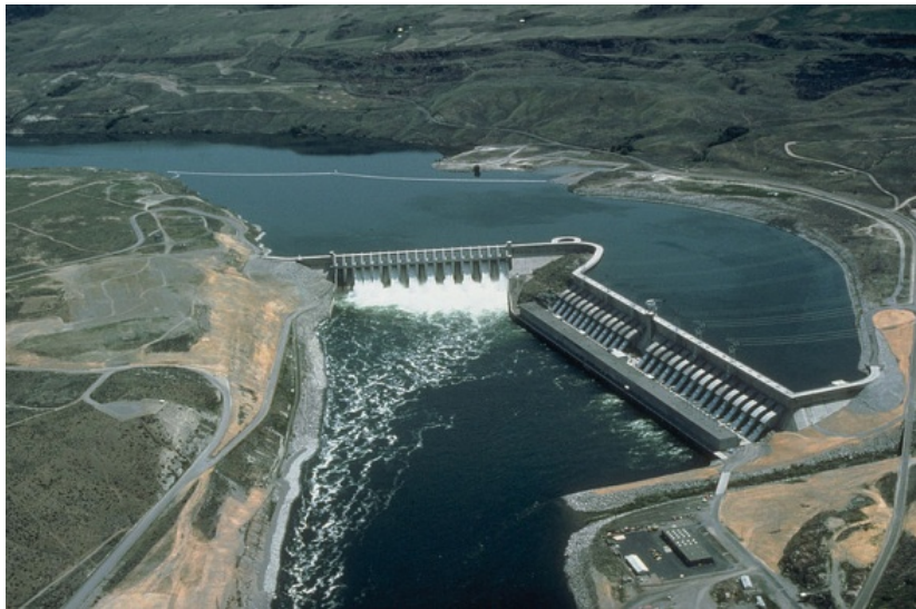
Figure 7.5-2 Chief Joseph Dam a Run-of-the-River Hydropower Plant (USACE 2010a)
