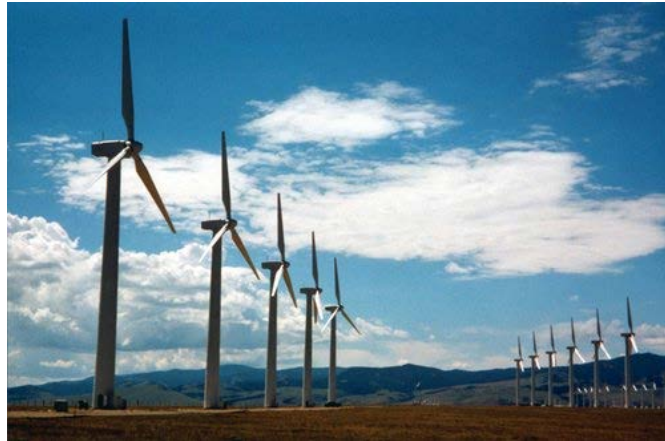
Figure 7.2-2 Wind Turbines at the Foote Creek Rim Project near Arlington, Wyoming (NREL 1998)
