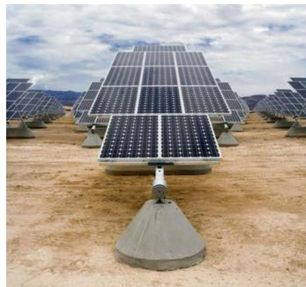
Figure 7.1-9 Photovoltaic Solar Power System at Nellis Air Force Base (NREL 2007b)
