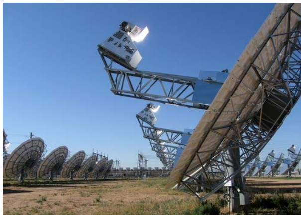
Figure 7.1-7 SunCatcher Solar Dish Engines at the Maricopa Solar Power Plant (NREL 2010c)
