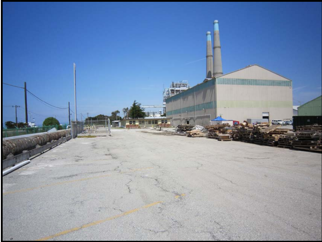
Photo Point 3: Highway 1 and select MLCC features, from MLCC site; view north. Highway 1 is left of pipe and fencing, in left portion of photo.
