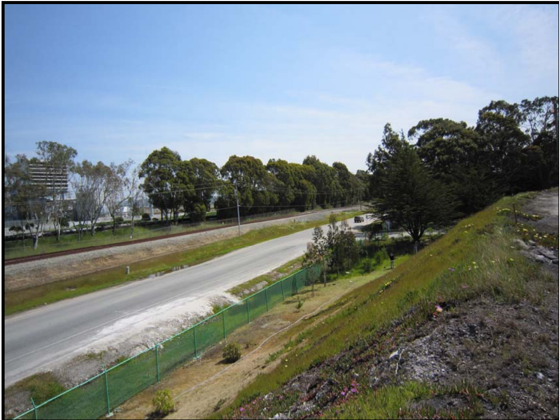
Photo Point 6: Dolan Road from MLCC site, north end of site; view northeast. Dolan Road, rail line, utility line, Moss Landing Energy Facility, and MLCC site landscaping visible.
