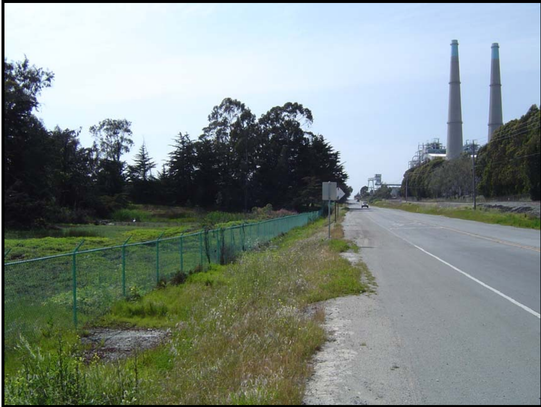
Photo Point 5: MLCC site from Dolan Road, northeast of site; view west. MLCC site obscured by trees; Moss Landing Energy Facility features visible to right.
