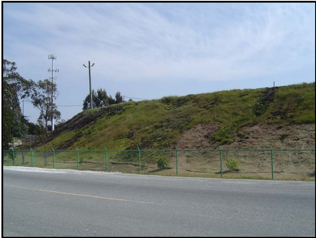
Point 20: Proposed aggregate laydown area from Dolan Road; view southeast.
