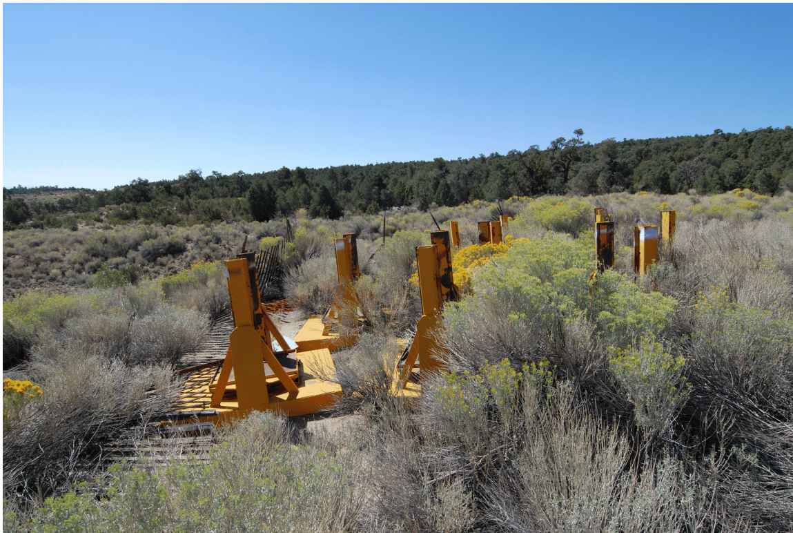
Figure 138. Plan map and photograph of Feature 79, U12t Tunnel, view south (2007).
