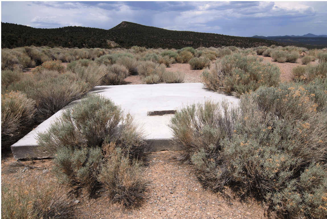
Figure 132. Plan map and photograph of Feature 73, concrete pad covering post-shot drill holes U12t.04PS#1A and U12t.04PS#1AA, U12t Tunnel, view northwest (2007).
