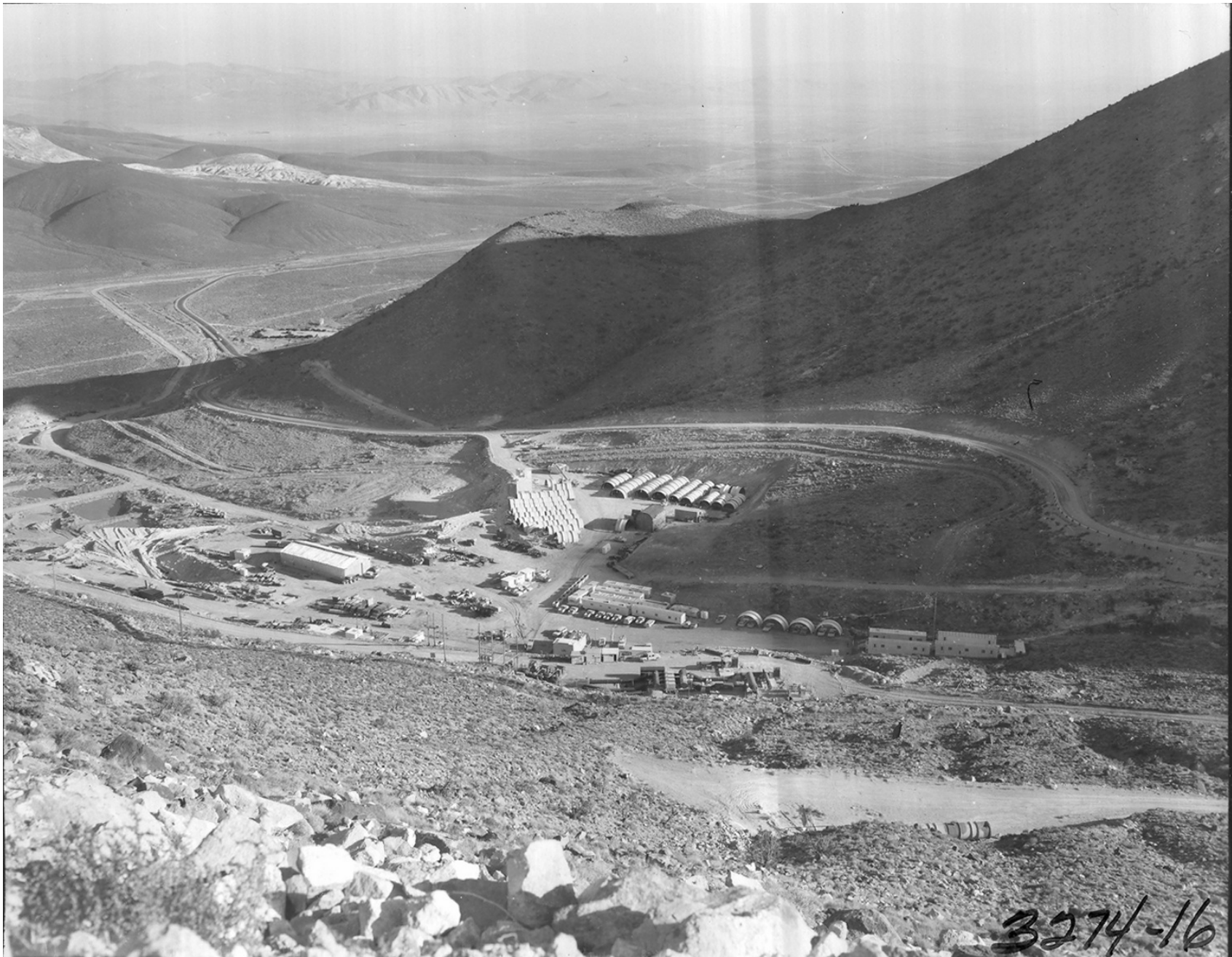
Figure 153. U12t Tunnel Portal Area, with storage of the half sections of the line-of-sight pipe for the Diamond Sculls test, view southeast, 1970 (photograph on file, Nuclear Testing Archive, Las Vegas).
