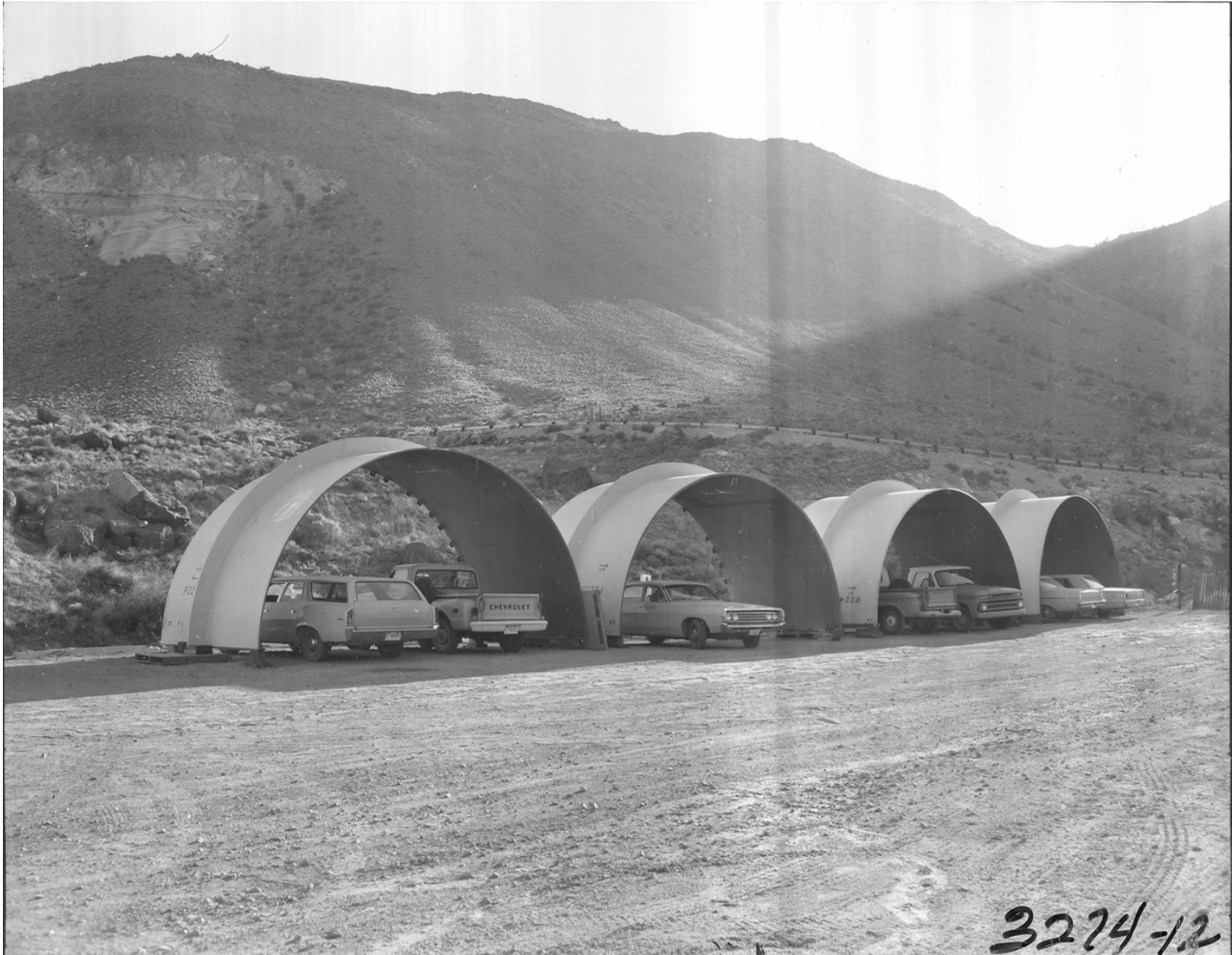
Figure 154. Half sections of the line-of-sight pipe for the Diamond Sculls test, U12t Tunnel Portal Area, view south, 1970 (photograph on file, Nuclear Testing Archive, Las Vegas).
