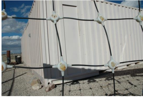
Figure 4. Netting Support Structure Connections.
