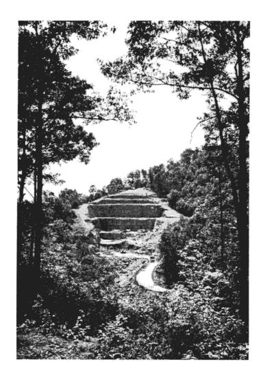
Figure 3.17-5. View north of the experimental excavation for the spillway, R. D. Bailey Lake Project (photo taken on July 5, 1973, Bechtell 1975).
