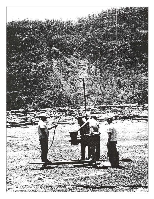
Figure 3.7-5. Drill rig and crew working on the crater floor after the Kilauea Iki Lava Lake had cooled enough to form a crust (Rawson and Bennett 1961, Figure 4).
