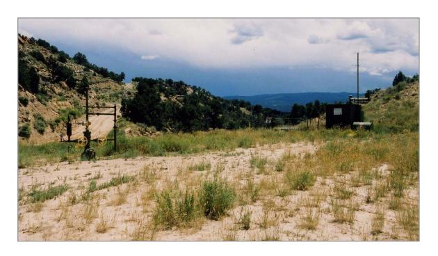
Figure 3.4-13. The DTU 25-11 well site. The well head is on the left in the photo and the monitoring shed and pressure relief pit are on the right (photo taken August 2005 on file at Desert Research Institute).
