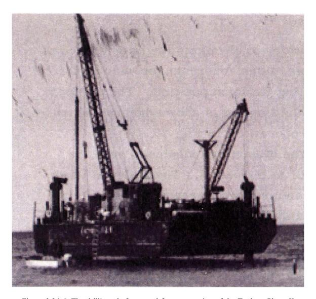
Figure 3.24-6. The drilling platform used for construction of the Tugboat Phase II emplacement holes (Day 1972, Figure 20).
