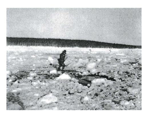
Figure 3.10-3. View of Operation Breakup yield scaling shot, Shot 31- a 940 pound charge was used (Kurtz 1966, Figure 4.11).
