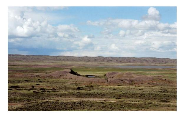
Figure 3.15-15. Project Pre-Gondola experimental row-charge trench at Fort Peck Reservoir, Montana. Because of an extended drought and a record-low water level, the 1,100 ft long trench is currently isolated from the reservoir (photo taken June 2004 on file at Desert Research Institute).
