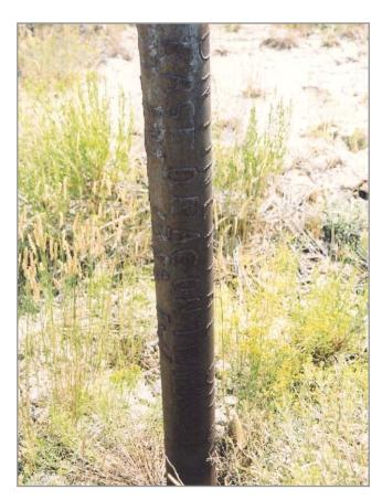
Figure 3.4-8. Close-up of welding on Project Dragon Trail study well DT-B (photo taken August 2005 on file at Desert Research Institute).
