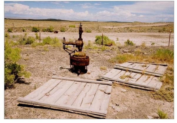
Figure 3.25-11. Drilling mud pit behind the Project Utah well head (photo taken August 2005 on file at Desert Research Institute).
