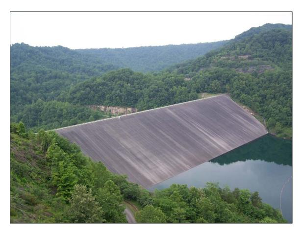
Figure 3.17-6. View of the upstream concrete face of the dam for the R. D. Bailey Lake Project. The spillway is located on the northern (far) side of the dam (<a href="http://en.wikipedia.org/wiki/R.\_D.\_Bailey\_Lake">http://en.wikipedia.org/wiki/R.\_D.\_Bailey\_Lake</a>, last accessed August 2008).
