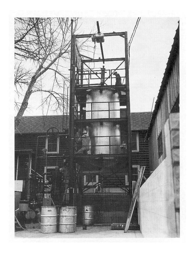
Figure 3.1-5. U.S. Bureau of Mines/ U.S. Atomic Energy Commission above ground experimental oil shale retort at the U.S. Bureau of Mines Petroleum Research Center, Laramie, Wyoming (Lekas et al 1967, Figure 5).
