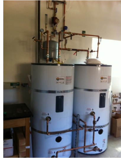
Figure 22. Twin 120-gal. water tanks within the REEF Workshop, used to store potable water under city pressure.
