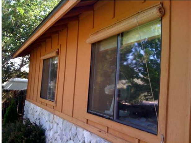
Figure 1 – Two west facing windows with bamboo blinds rolled up
