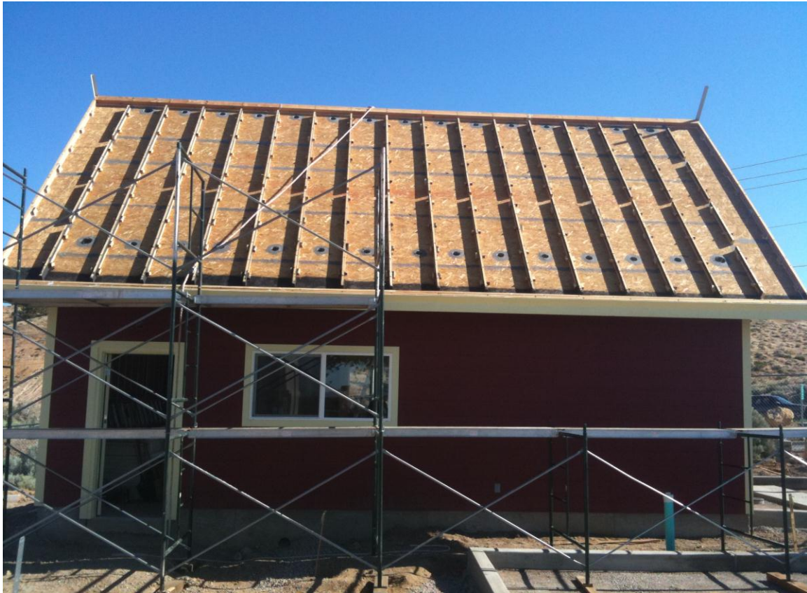
Figure 5 Completed Roof Collector Framework Ready for Absorber and Glazing
