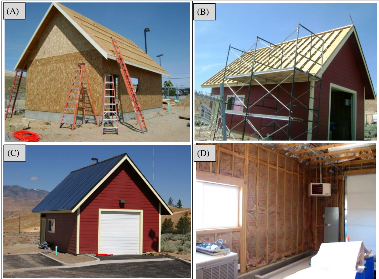
Figure 5. Photos of DRI-REEF Workshop Construction.
