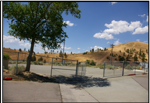
Figure 2. Photo of DRI-REC (REEF) site before start of construction.
