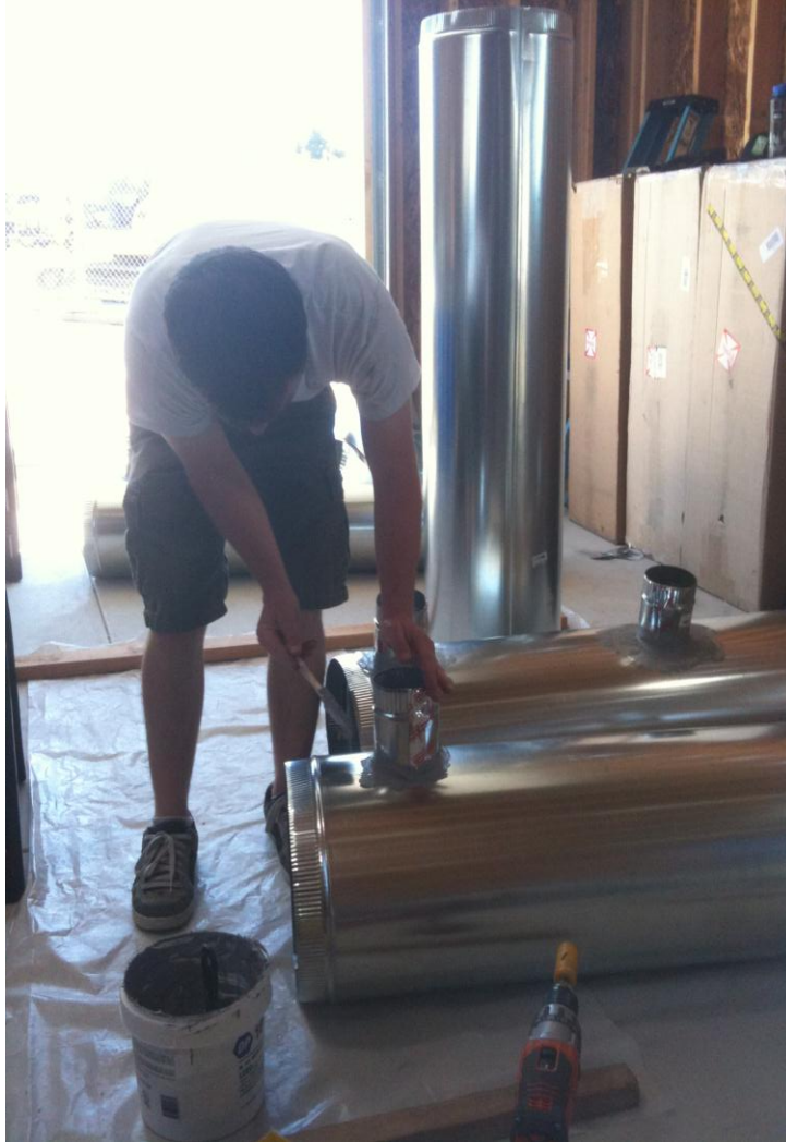
Figure 10 A 4" diameter collar is screwed then caulked to the 14" diameter header. The header ducts are then assembled in place with the collars aligned to the collector collars inside the roof. Corresponding collars are then connected with flexible ducting.
