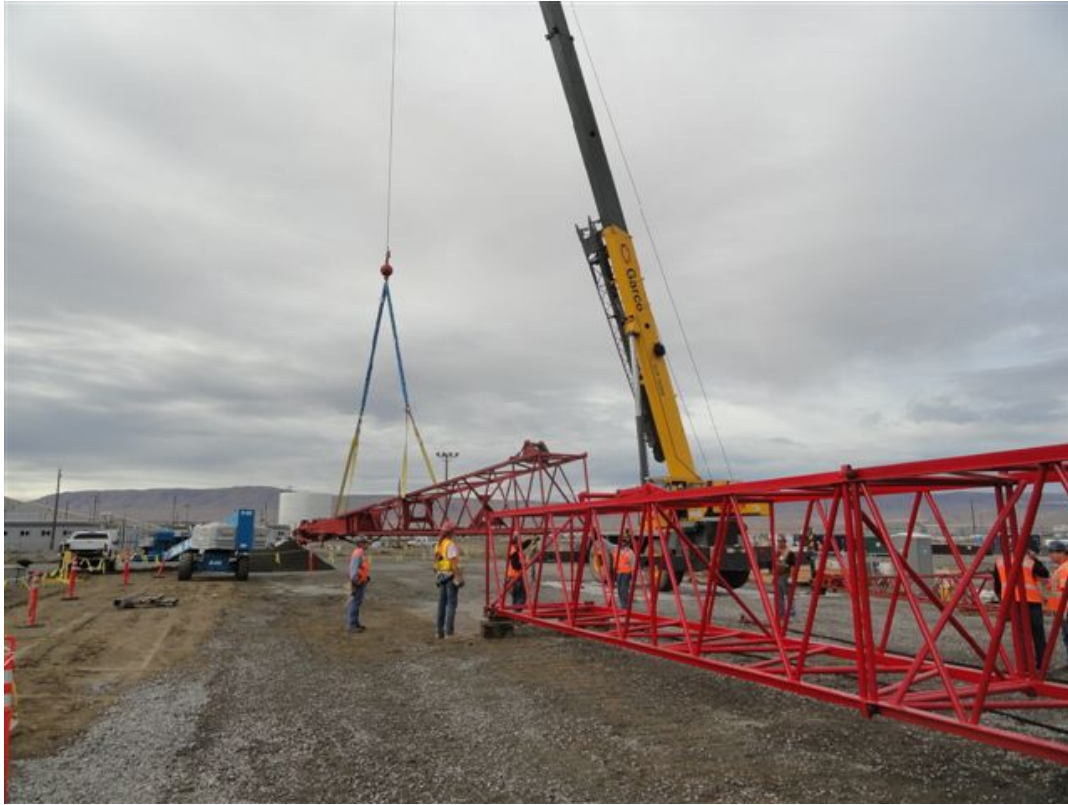
Figure 6 - Assembly of 100-Ton Crane at 2W P&T
