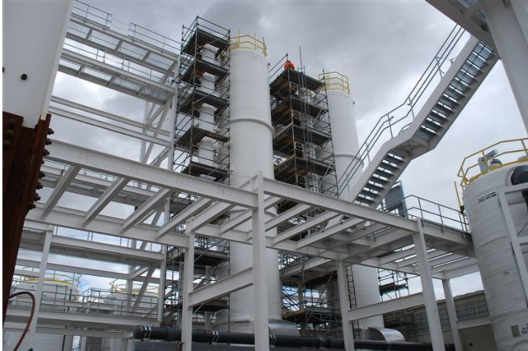
Figure 12 - Scaffold Erection at the Air Stripper Towers at 2W P&T
