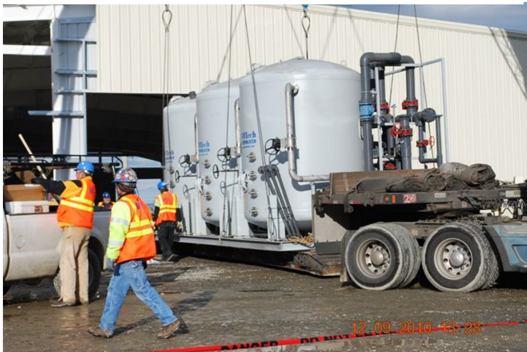
Figure 7 - Delivery of Avantech® IX Tank Skid for the 2W P&T Project
