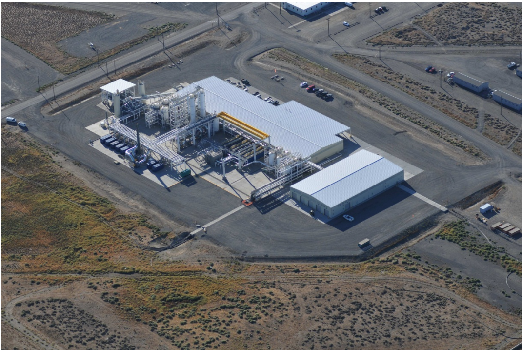
Figure 3 - 2W P&T Facility
