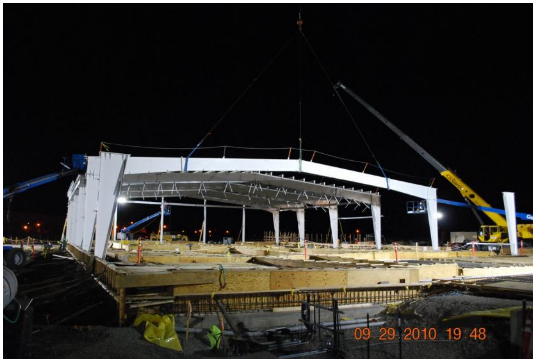
Figure 11 - Steel Erection of Rad Building at 2W P&T
