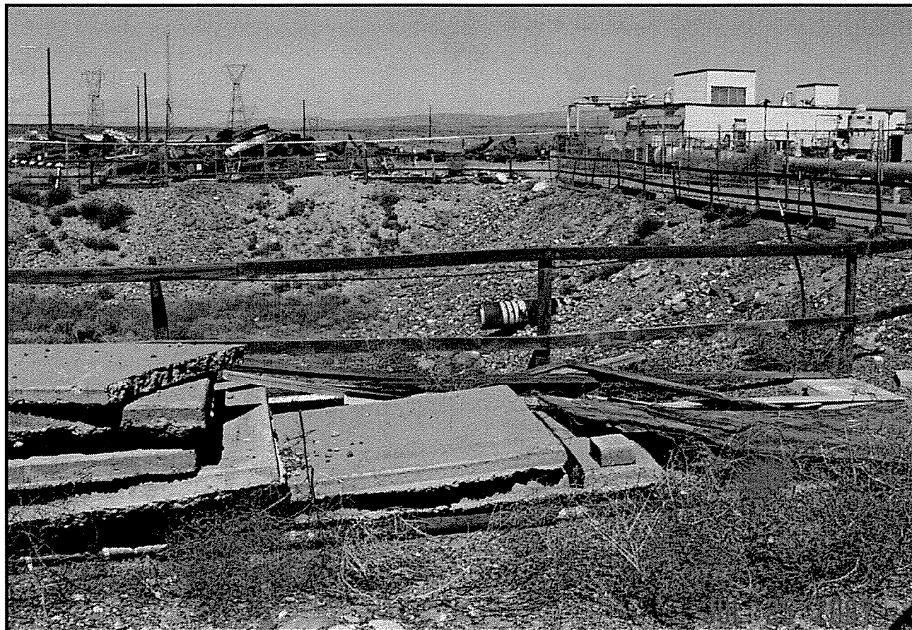
Figure 5. 183-ND Resin Disposal Pit.
