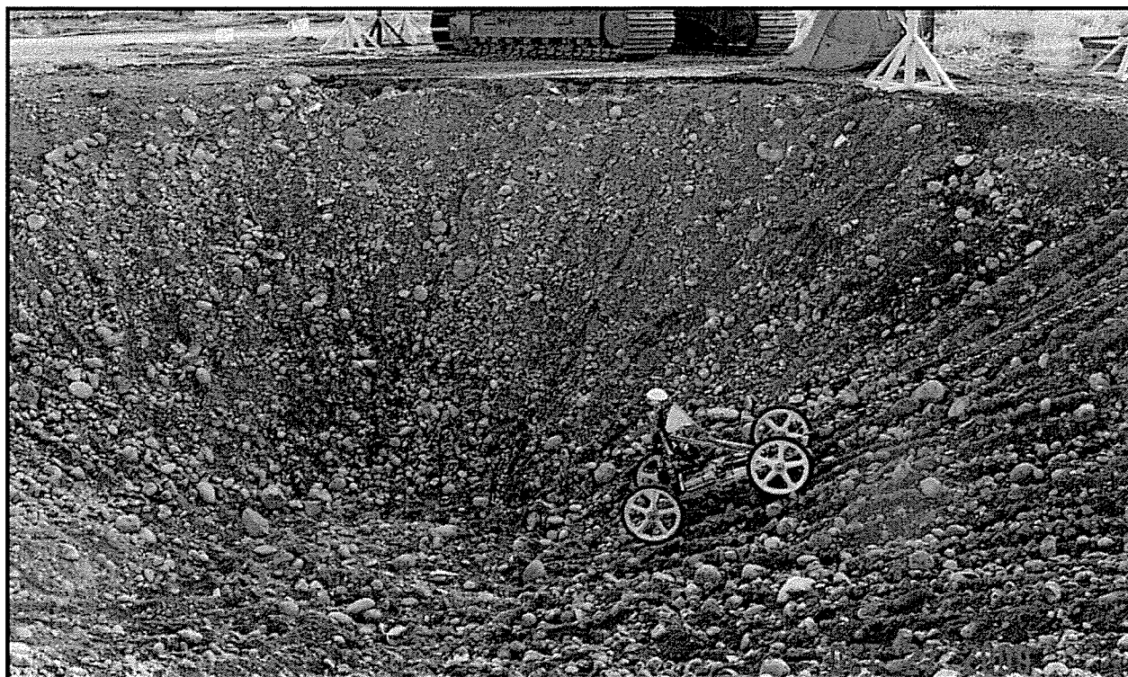
Figure 12. 1706-NA Sewage Lift Station Excavation.
