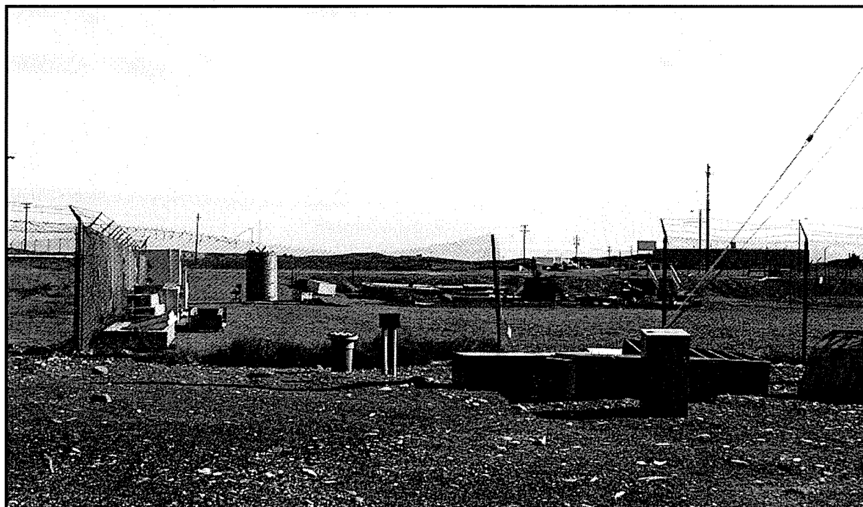
Figure 9. 1525-N Laydown Yard in 2006.
