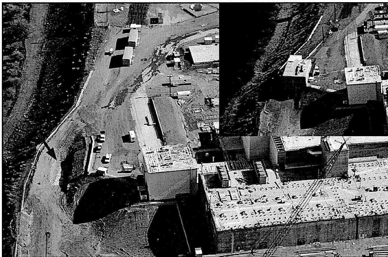
Figure 3. Post-Demolition Condition of 107-N; Inset Shows Original Structure.
