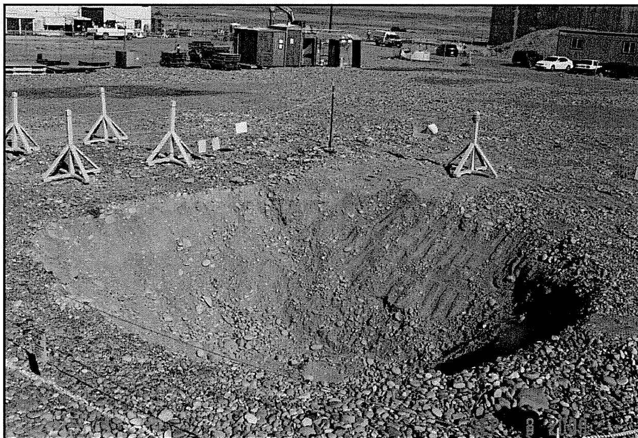
Figure 10. 1607-N1 Tank Excavation.
