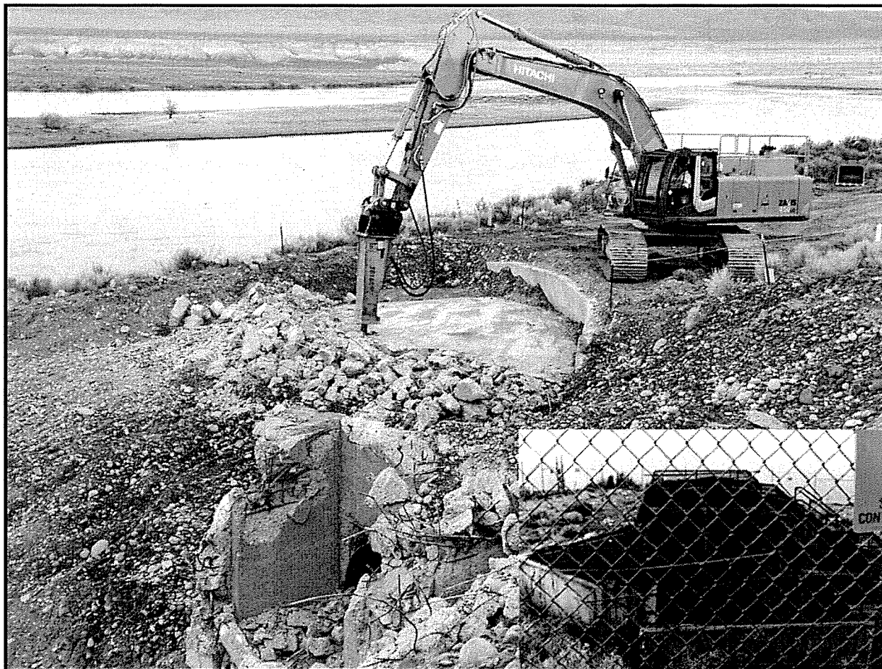
Figure 13. Demolition of the 1904-D Outfall Structure; Inset Shows Original Structure.
