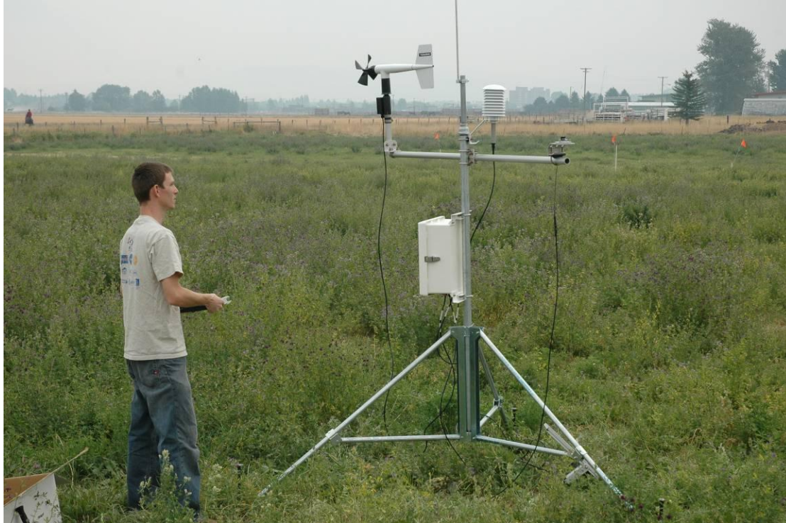
Figure 19. Solar-powered weather station being installed at the ZERT field site in Bozeman, Montana in September 2006 (the solar panels are not yet installed here)
