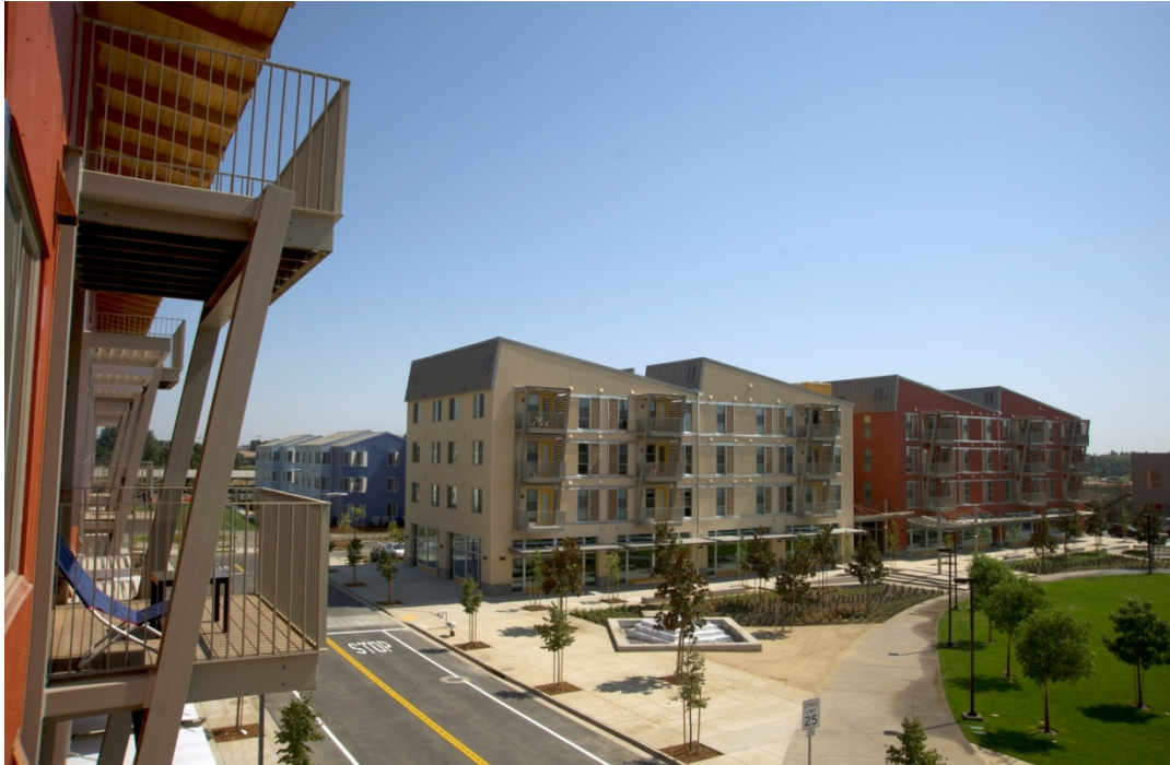
Figure 1. Photograph of the completed village square surrounded by mixed use and student housing buildings
