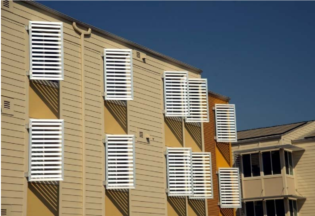
Figure 2. Exterior window sunshades on the student apartment buildings
