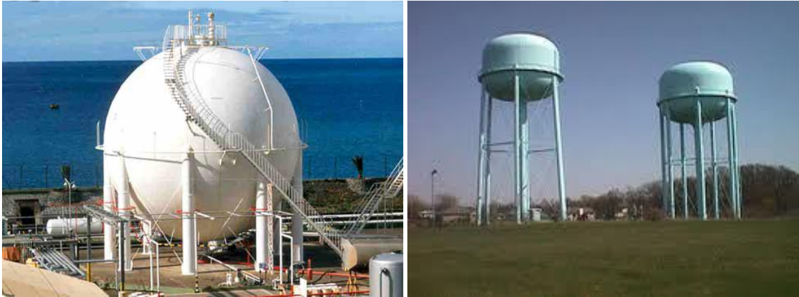
Figure 5. Butane Storage Tank and Water Towers with Legs
